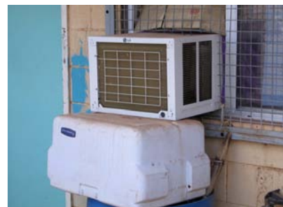
TAN3- poorly installed in-window air conditioning systems removed
