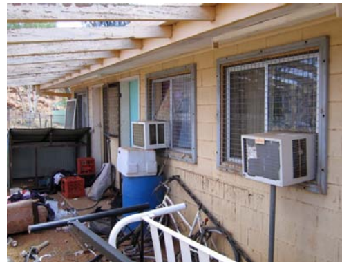
Tan3 existing in-window reverse cycle (heating & cooling) air conditioning systems x4 before thermal upgrades (removed after installation of new cooling system)
