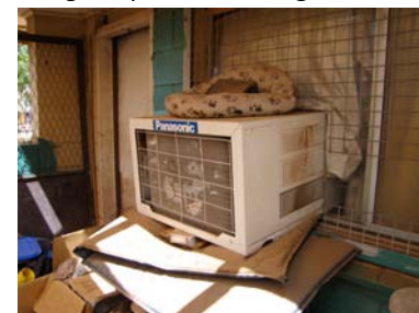
Reverse cycle air conditioning- active cooling (used before thermal upgrades)
