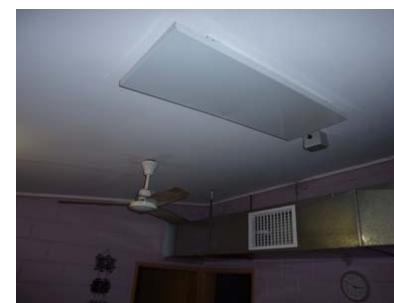
new ceiling mounted radiant heaters, new evaporative cooling system ducting, ceiling fan- active cooling
