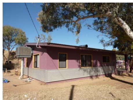
House Tan 2 after thermal upgrades - new evaporative cooling system, new shade wall
