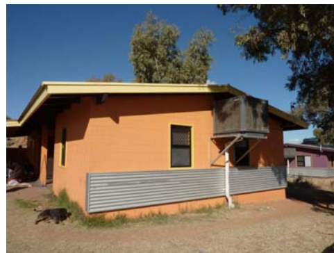
House Tan 1 after thermal upgrades west elevation. New shade wall, new ducted evaporative cooling system, new pergola roof to north
