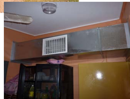
New evaporative cooling ductwork
