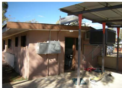
Tan3 new ducted evaporative cooling system
