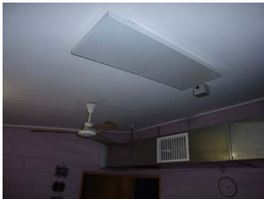
new ceiling mounted radiant heaters in bedrooms, kitchen & living, new evaporative cooling system ducting, existing ceiling fan
