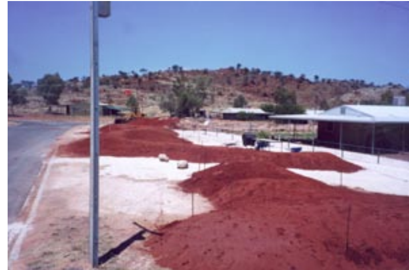
6. View of the completed first mound and the beginning of the second at Pipalyatjara. Note the drum oven which was used to cook evening meals, adjacent to the floor of the first mound. [October 2000].
