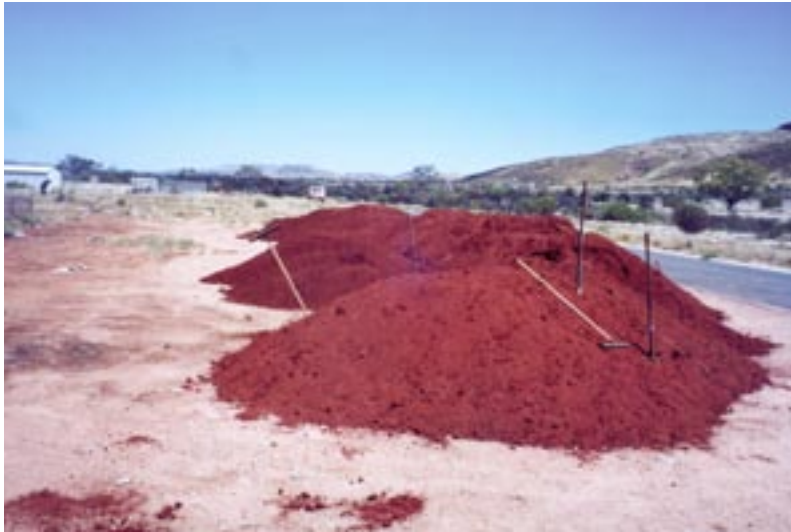
5. View of soil which has been tipped along a centre line, thus determining the general shape of the mound. Note the half loads of soil on the inner side of the mound which will be used to form the floor [October 2000].
