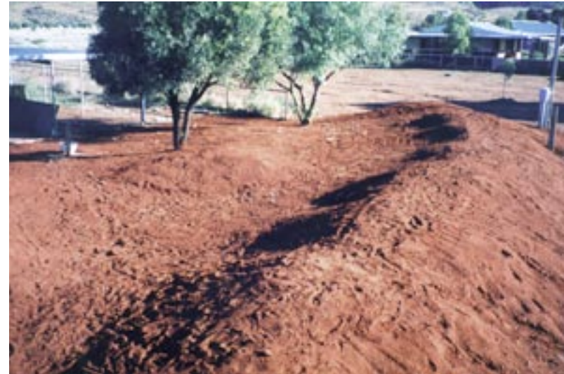
22. View of part of the mound system which has been shaped from the soil in picture 21. Note the outer primary mound and inner secondary mounds which flow in around the trees to the front veranda [August 2001].
