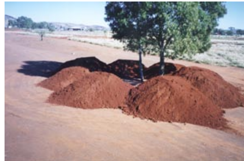
8. View of an open compacted area at Kalka which has been eroded. Soil has been tipped around these trees and when shaped, will collect some of the storm water run-off [August 2001].
