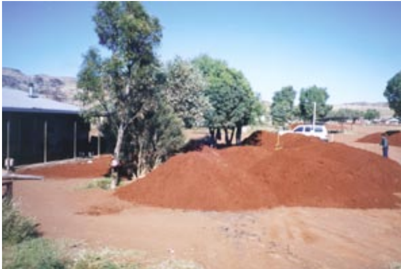
21. View of fresh soil which has been tipped in a crescent shape in a front yard at Kalka after the fence has been removed. An outer primary mound will be shaped to encircle inner secondary mounds [August 2001].
