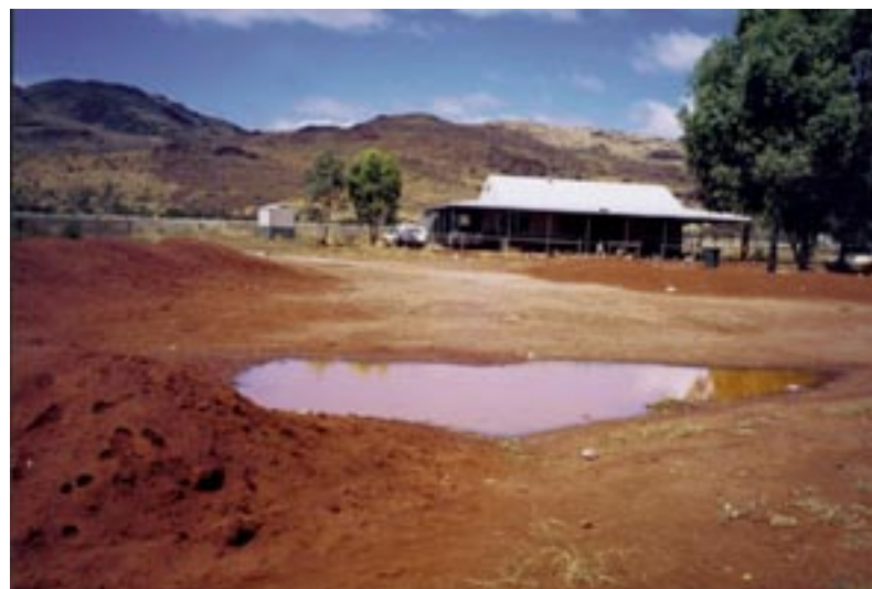
12. Mound systems are being built on open compacted areas to change the shape of the soil surface and collect storm water, thus preventing it from draining into the road system [October 2001].
