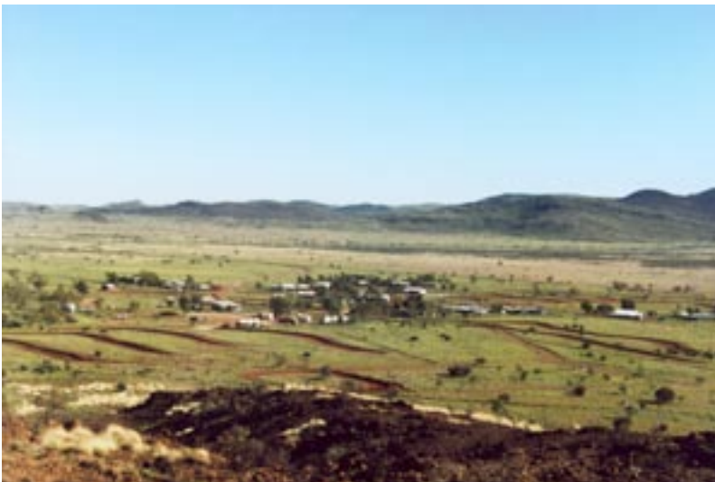
3. View of the ponding banks built from the top of the watershed to manage storm water, preventing it from entering the community road system [March 2001].
