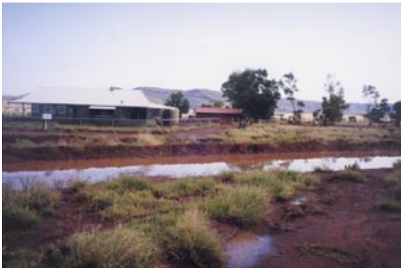
9. The storm water collected in this ponding bank, no longer floods through the house yard below it [October 2001].
