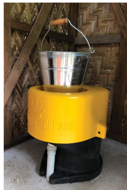
02 Pedestal Cap & 03 Urine Diverting Pipework
