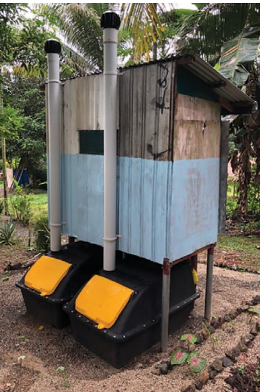
04 Dehydration Tanks & 05 Ventilation Pipework & Ventilators
