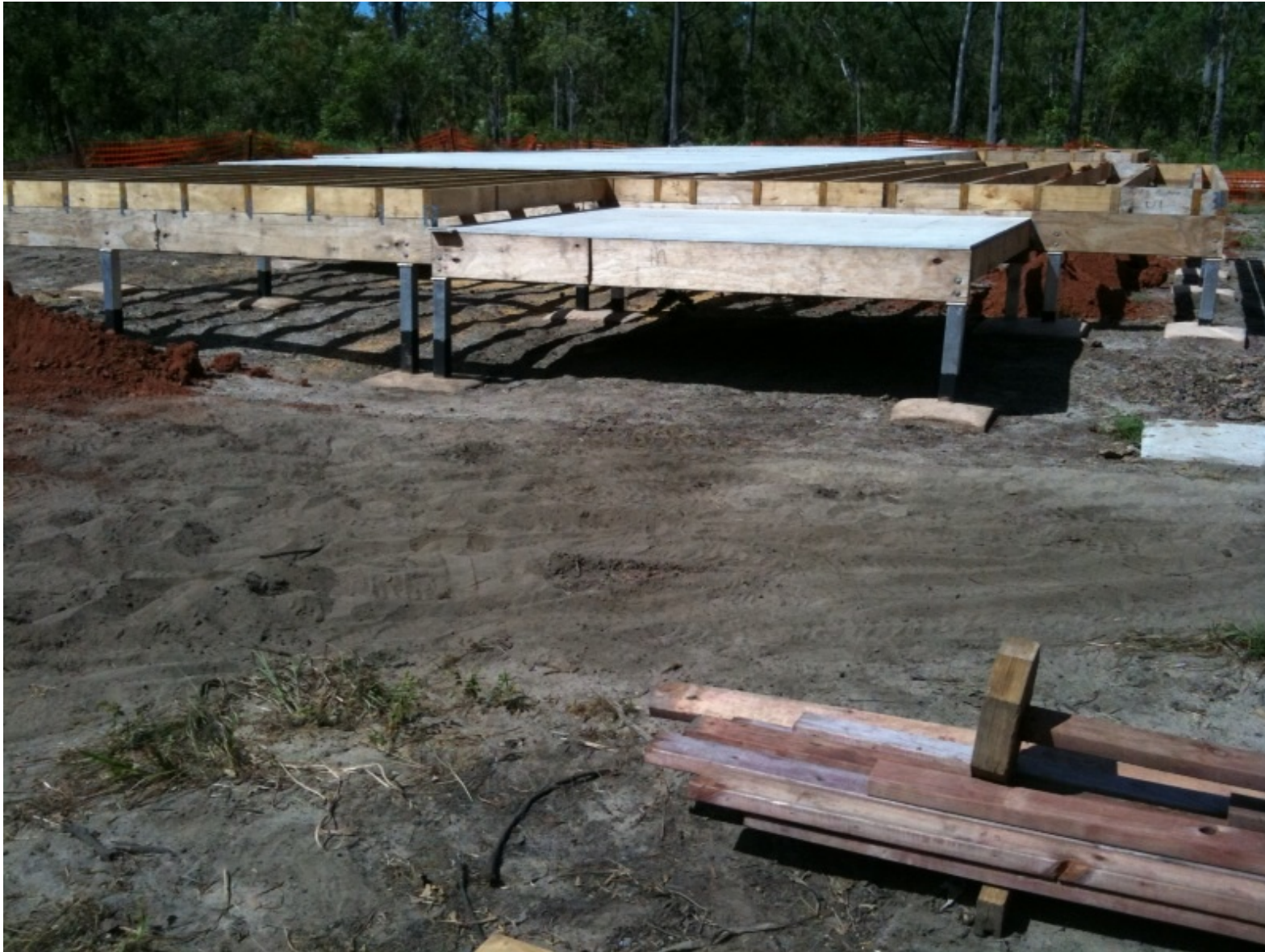
Subfloor construction in laminated veneer lumber (LVL) on “a northern community” 2009-10 (NIHG Safety structural safety)
