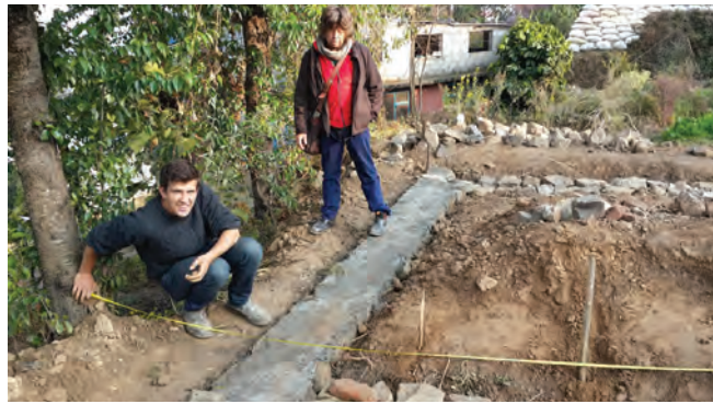
Measuring and siting existing footings.
