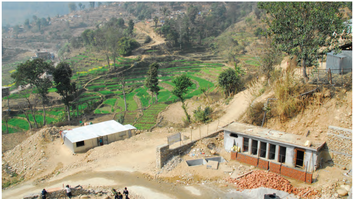
Boys toilet block and septic tank under construction (right) and village beyond
