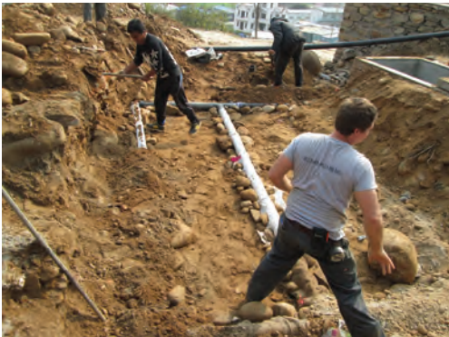
Soakage trench pipe work
