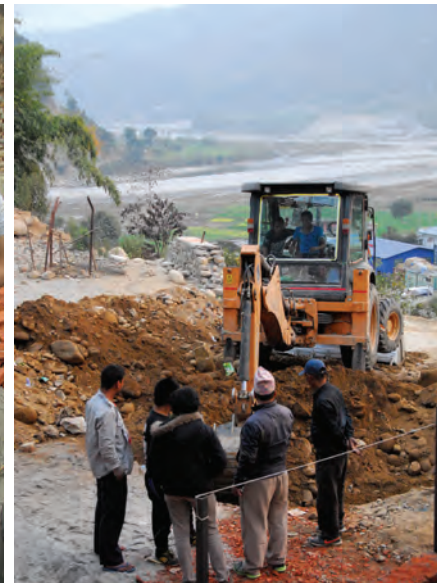
Excavation work for septic and soakage trench
