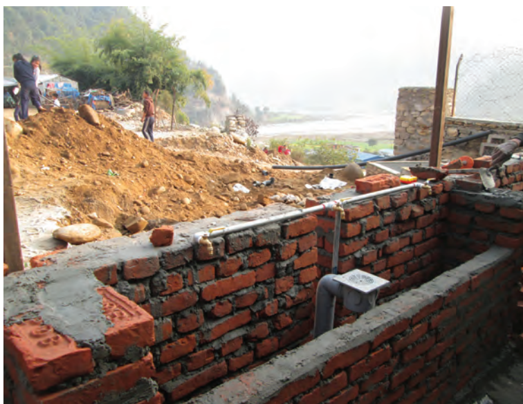
Structure for sink trough built around plumbing
