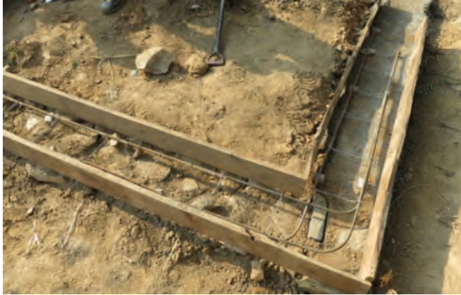
Seismic band formwork and reinforcement steel assembled onsite with local team to test construction method
