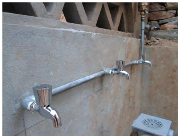
Taps and drain installed to toothbrushing sink
