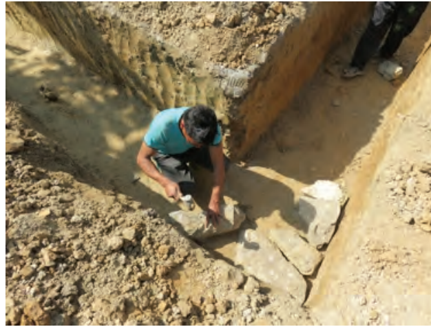
Laying first course in footings to prototype house
