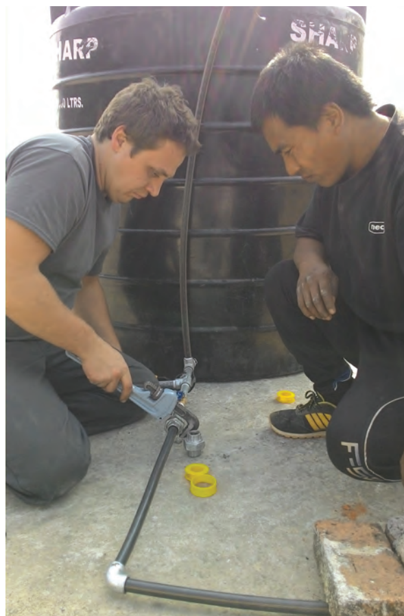
Water supply: Gravity fed from top of school to toilets.
