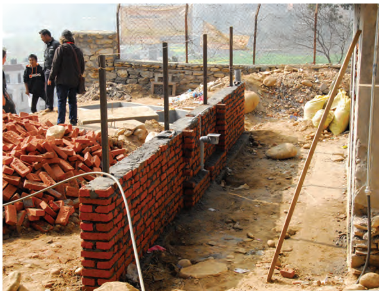
Taps and drain installed to hand-washing sink
