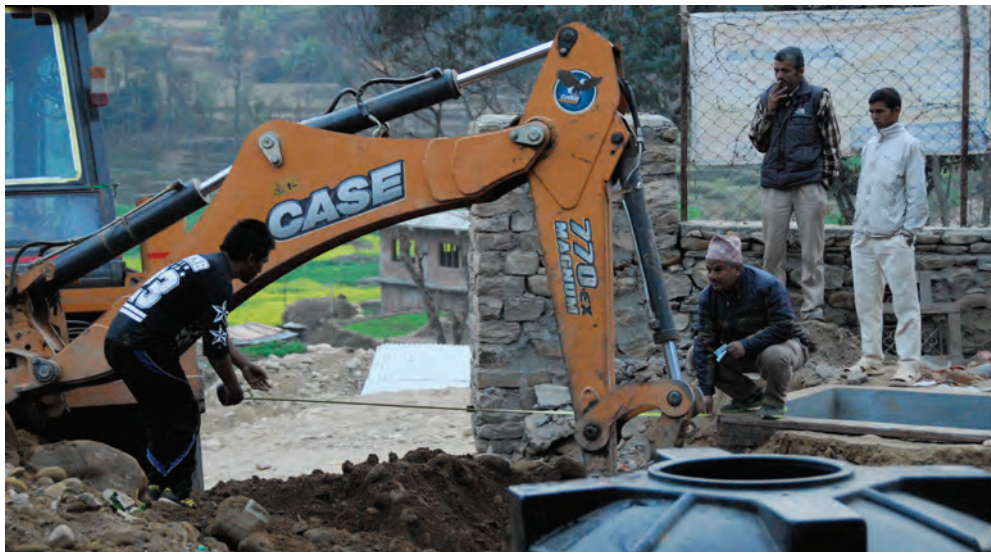
School principle (right) and local plumber Lok (left) setting out soakage trench off septic tank
