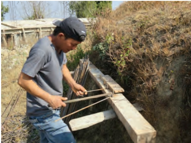
Local team set up an onsite jig for bending steel used for reinforcement in the seismic bands
