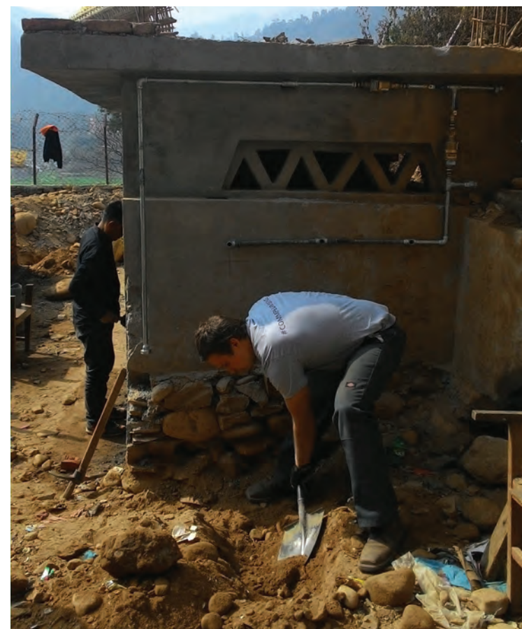
Ground preparation for drainage from toothbrushing sink
