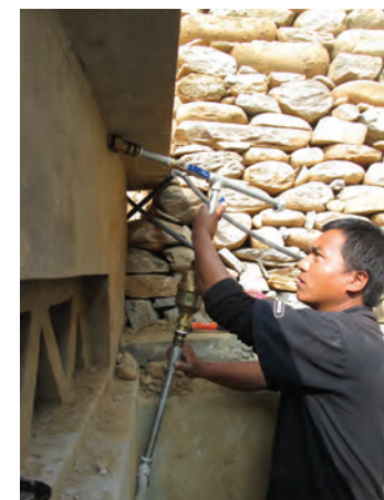
Water meter installed to toothbrushing sink
