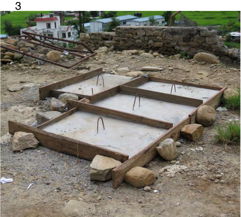
1 Main drainage line being set out 2 Setting out the pans and breaking through for plumbing 3 The septic tank lids cast on site 4 The trench for the effluent pipe from septic tank to soakage trench 5 Excavation of the soakage trench bed with connecting pipe trench
