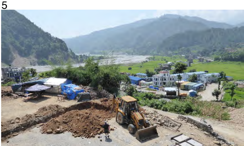
1 Main drainage line being set out 2 Setting out the pans and breaking through for plumbing 3 The septic tank lids cast on site 4 The trench for the effluent pipe from septic tank to soakage trench 5 Excavation of the soakage trench bed with connecting pipe trench
