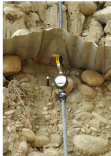
Meter to tap point installed during the visit
