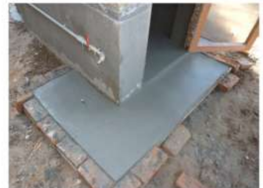
Toilet pan setting, toilet floor and spte with outside tap base work.
