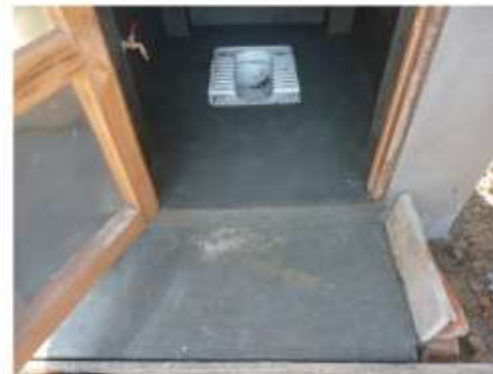
Toilet pan setting, toilet floor and spte with outside tap base work.
