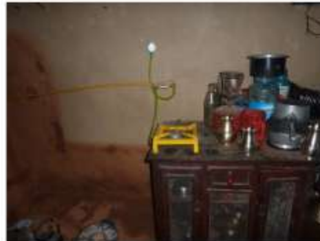
Under ground biogas work and gass stove installed in the kitchen.
