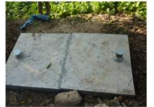
Under ground septic tank brick, slab, plumbing and cement cover.
