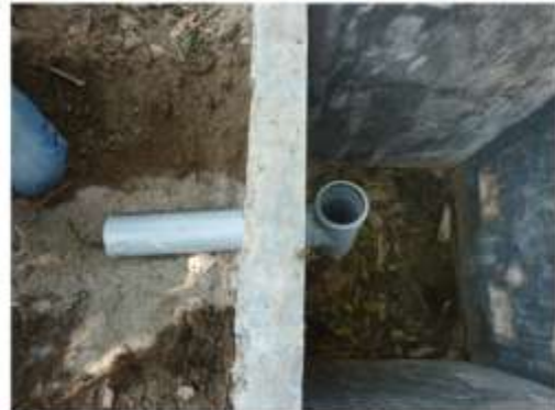
Under ground septic tank brick, slab, plumbing and cement cover.
