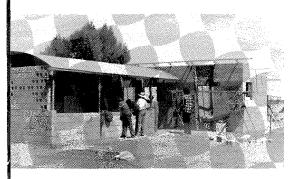
Figure 2 Renovation of a Kingstrand Hut (left) at Yuendumu in Central Australia. These transitional houses were built during the 1960s and are shown here being upgraded and extended during September 1987 to better suit community needs. [Source: AERC, University of Queensland. Photographer: P. Memmott.]
