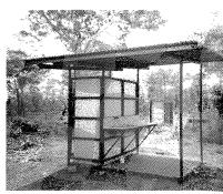
Figure 1 A drawing and photograph of a shower and laundry waste-water system designed by Build Up Design and installed in Arnhem Land outstations for the Bawinanga Aboriginal Corporation. [Photographer & Artist: S. Scally.]
