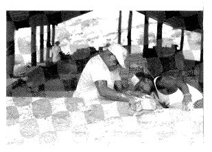
Figure 4 Hobson Levi shows the chairman of neighbouring Boigu Island how to lay mud bricks. [Photographer: P. Haar, 1987.]
