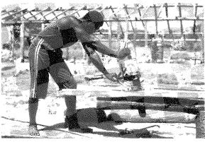
Figure 3 Robbie Ware mills window frame timbers from local mast-wood (Podocarpus greyii) using a chainsaw and simple 'Granberg Mini Mill' attachment, St Pauls. [Photographer: P. Haar, 1987.]
