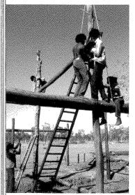
Figure 1 Previous work experience at Top End cattle stations had equipped the Mt Catt mob for the challenge of hoisting heavy pole timbers into the roof structure. [Photographer: P. Haar, 1987.]
