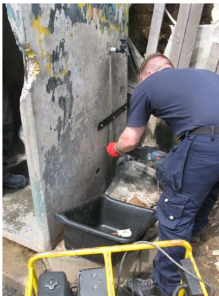
LEFT measuring the correct height for the washing tubs , CENTRE fitting the tubs
