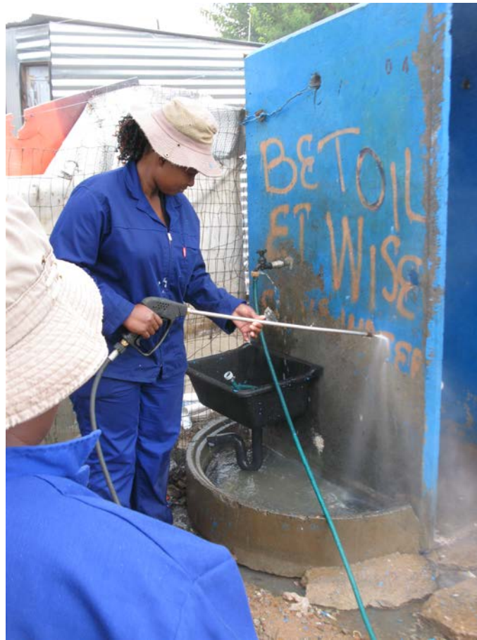
CENTRE high pressure water cleaning and wall patching
