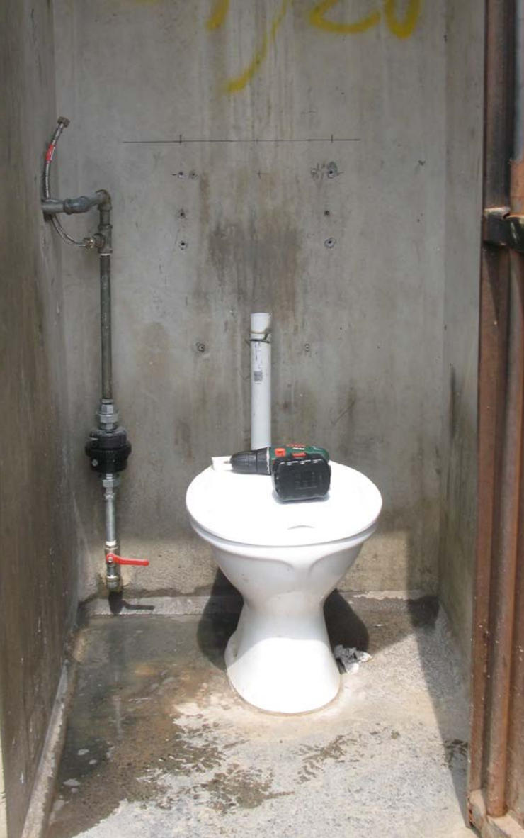
LEFT pan awaiting new cistern, water shut off
