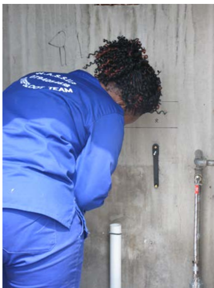
CENTRE fitting the flush pipe and fixing brackets
