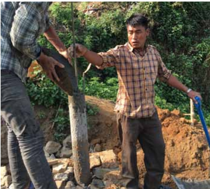
4" core hole pipe being lifted as concrete filling in hole
