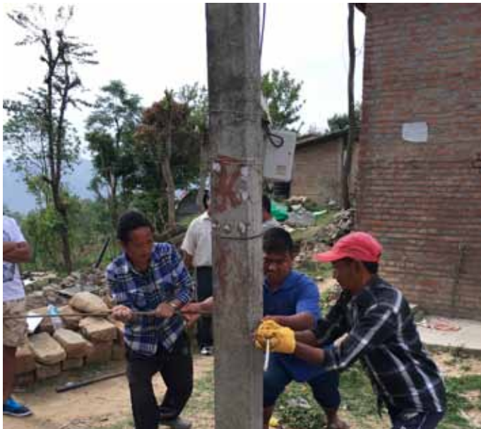
Using a concrete power pole in the village to bend the steel for L's and T's in a consistent fashion
