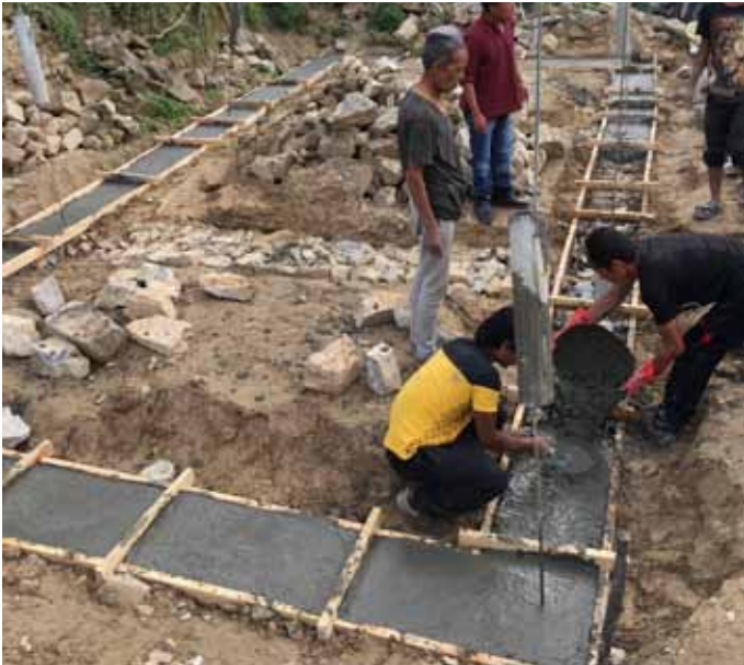
Pouring concrete into band 1 formwork
