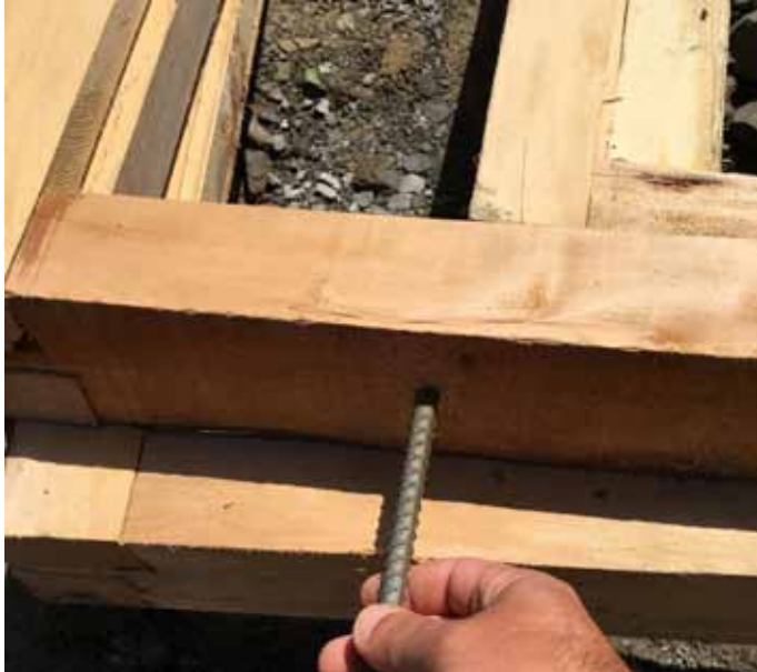
"Hold pass" being installed in the window and door frames
