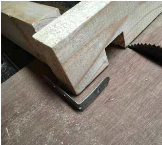
1 1/4"x3" pine formwork for banding made offsite by carpenter Triratna. Nails better then brackets as no screw drivers not available onsite.
