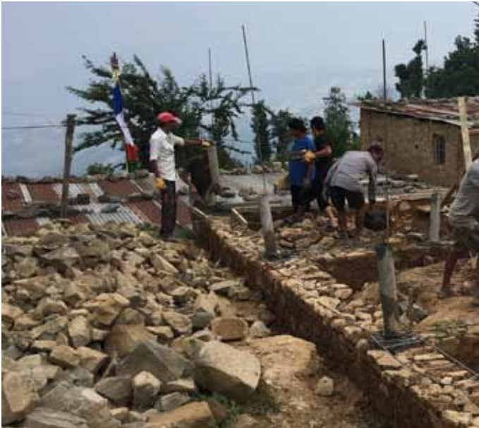
Banding team setting up L and T reinforcement at corners and cross walls
