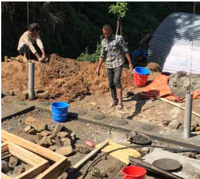
Attempt to make clumps when concrete band set did not bind to band adequately
