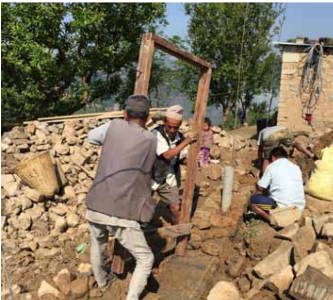
Door supplied and located by the household following simple rule of allowing a 4 1/2' offset from outside face of stone work to door jamb
