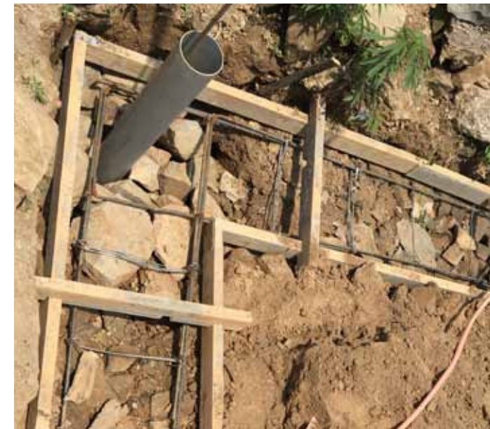
Ensure 3x 3mm wire at L's and T's
