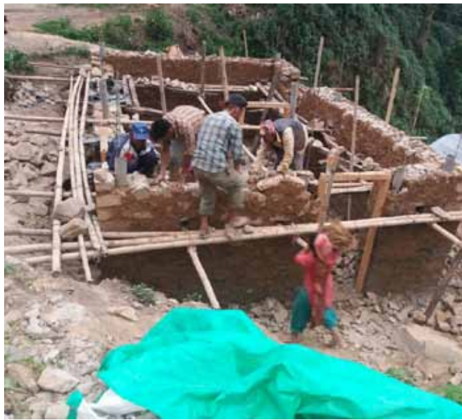
Bamboo scaffolding in place and stone masons progressing to 6' band
