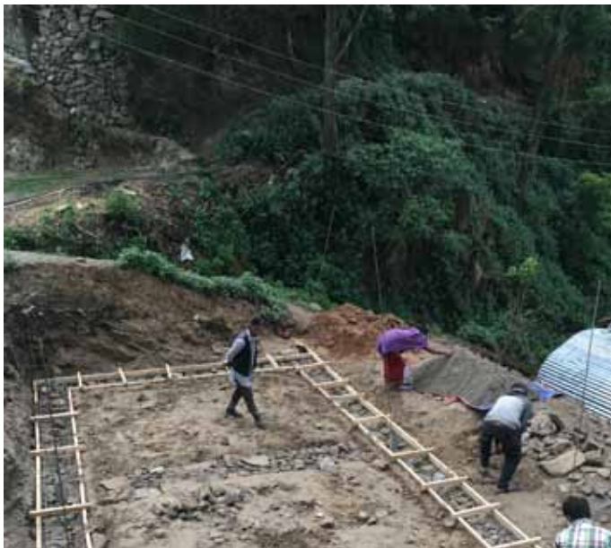
3"x1" timber formwork for banding laid in place for 3"x1" cross pieces
