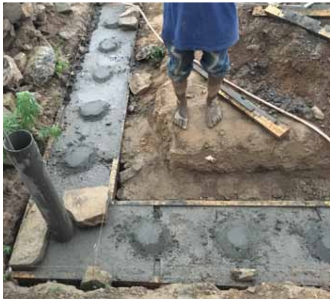
Sand and cement clumps at 1' spacing to be applied to wet concrete or mortar in every case
