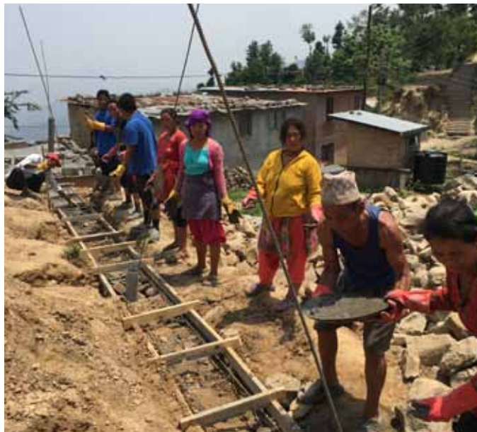
Unskilled labour assisting with a human conveyor belt passing concrete from batching to band
