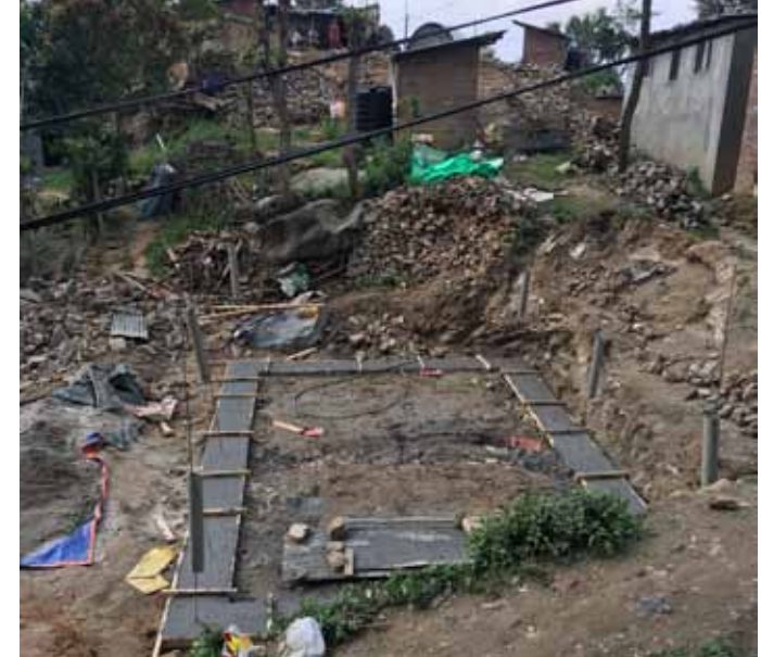
The completed first band at foundation level : 6 bags cement used to this point
