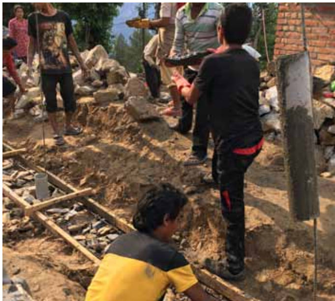
Banding team installing reinforcement and formwork for band 1
