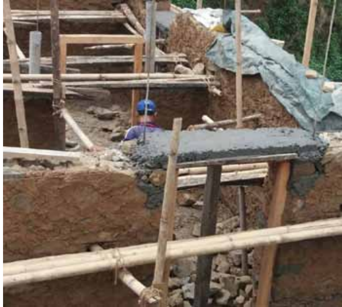
Concrete lintel laid over door
