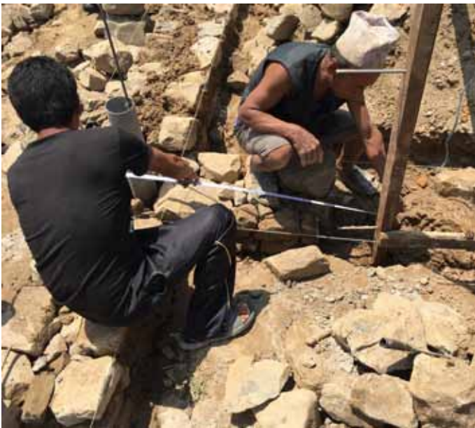
Checking for 4 1/2' offset minimum, allowing for T reinforcement
