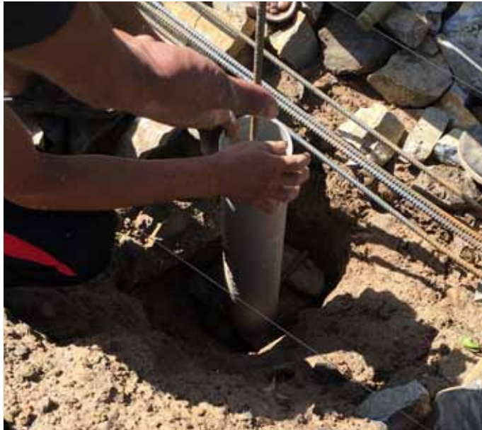
Placing cogged vertical bars into holes and replacing stone around tightly
