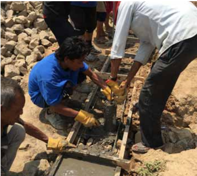
Filling 4" PVC pipes with concrete
