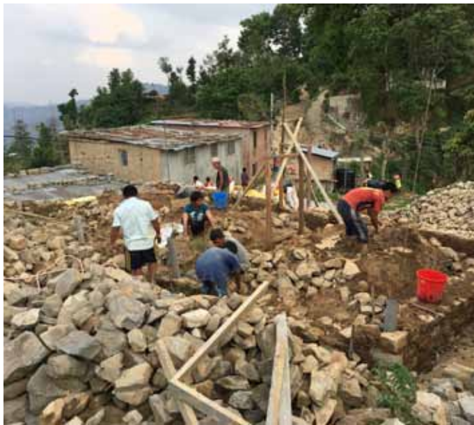
Stone mason team building up first 2' level of wall
