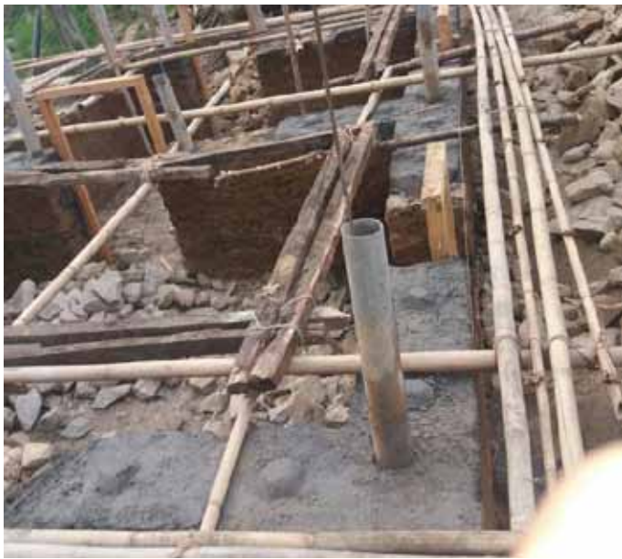
Clumps shown on wet mortar L's and T's - photos by Surya Tamang
