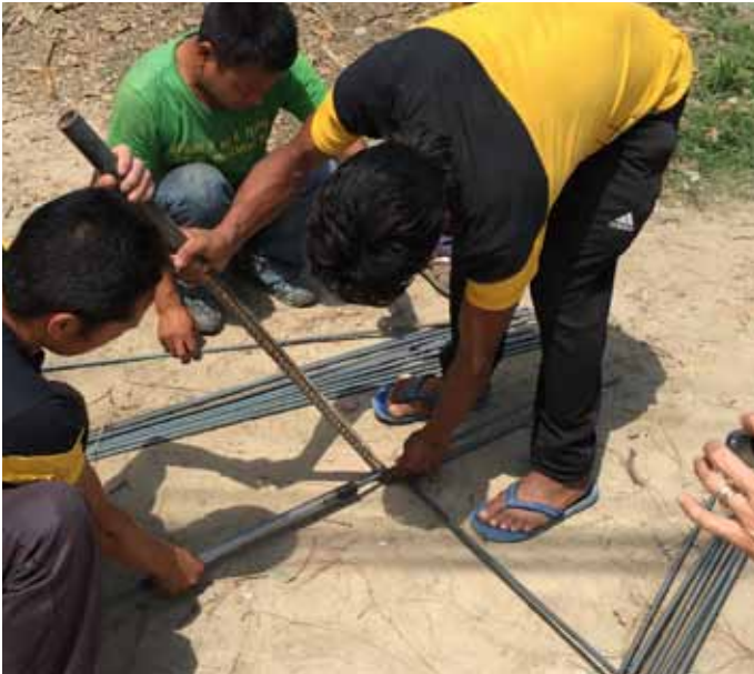
Banding team bending the L's for band 1
