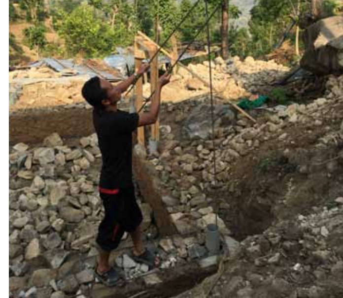
L reinforcement being threaded over vertical reinforcement
