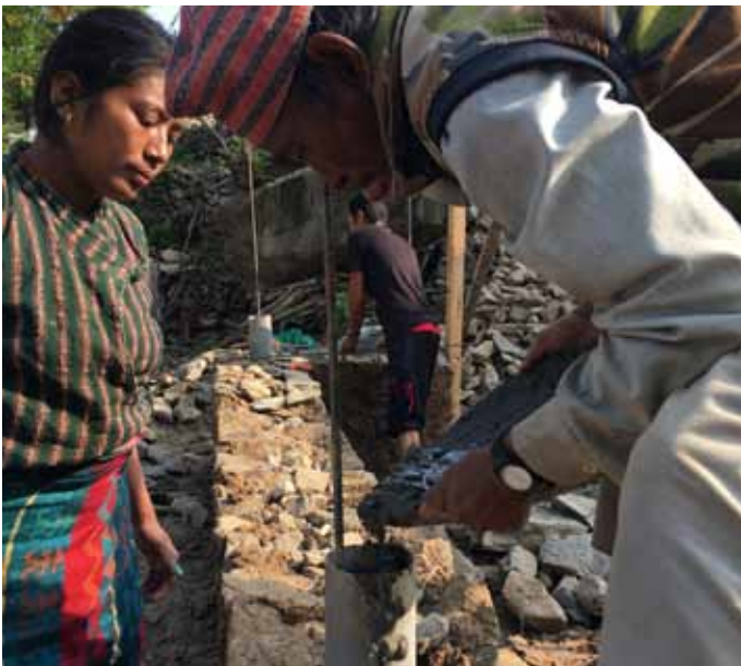
2' band level, vertical rod core holes being poured
