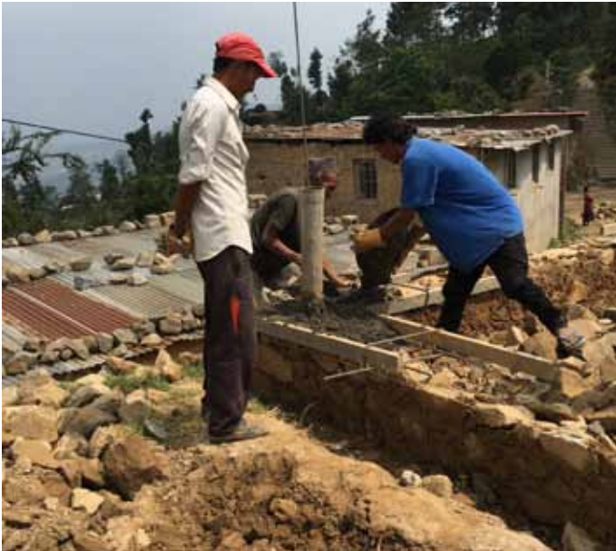
Banding team pouring mortar to L's and T's
