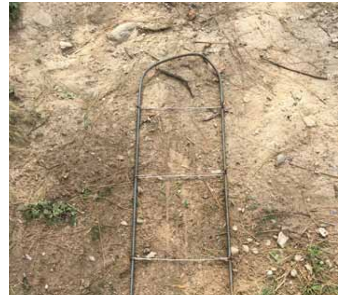
Completed component of L and T reinforcement ladders
