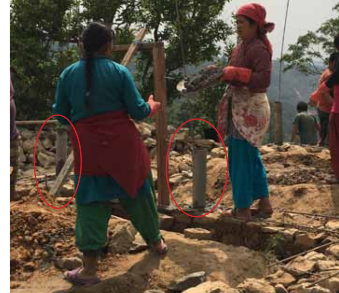
Ensure 4" pipe and vertical rods are located at all door jambs during the first stone course
