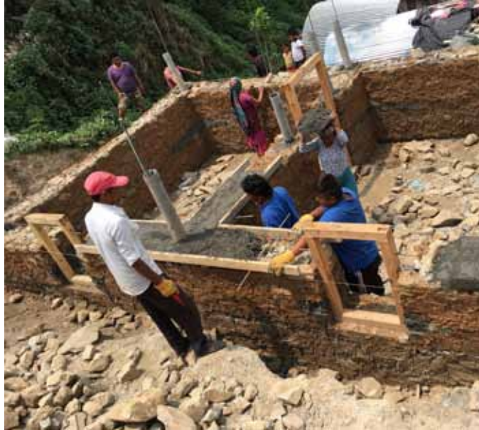
Mortar mix being poured at T and L junctions
