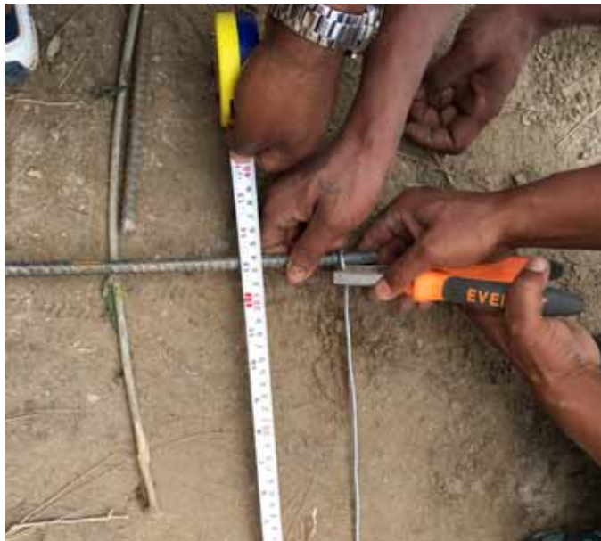
Closing 3mm wire ties securely around the 10mm rod to prevent it slipping out of place
