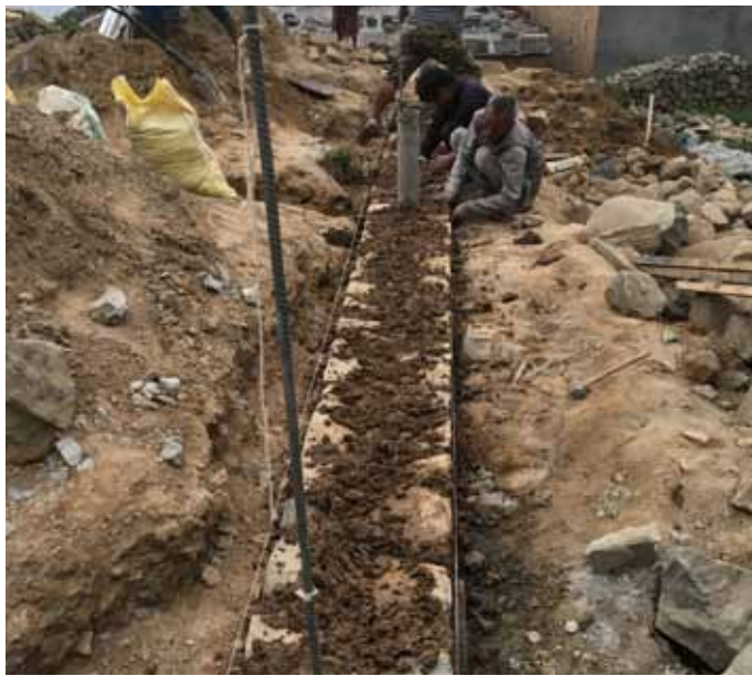
Local mud placed onto stone to secure the next course
