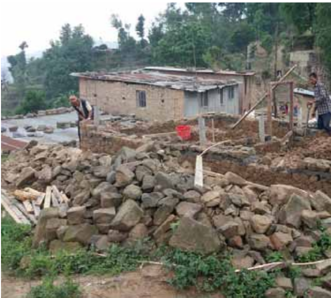
Stone masons progressing following completed 2' banding - photos this page by Surya Tamang the next week
