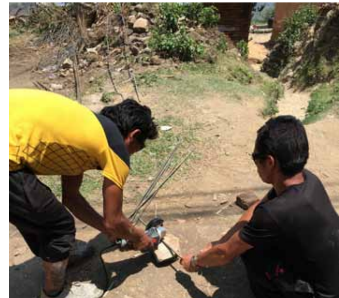
Angle grinder was essential for cutting 10mm steel reinforcement bar - gloves and protective eyewear were also essential
