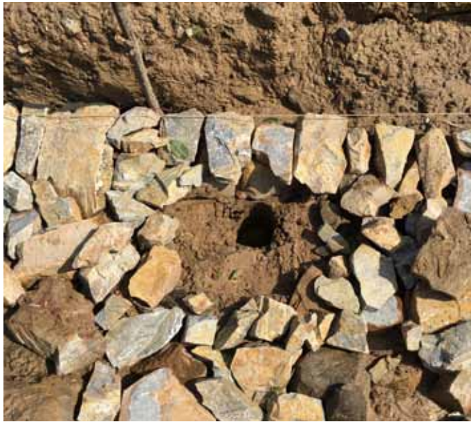
Issues found with junctions at cross walls and corners not dug to allow for 4" pipe and rod
