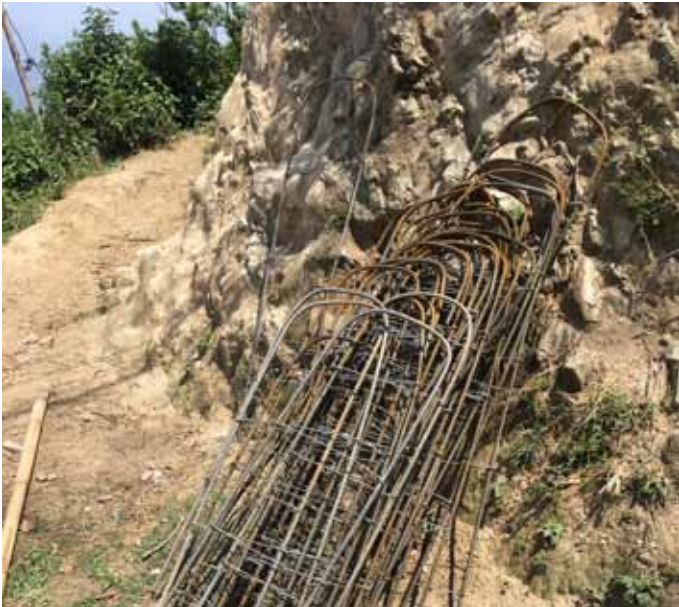
Completed L and T reinforcement ladders
