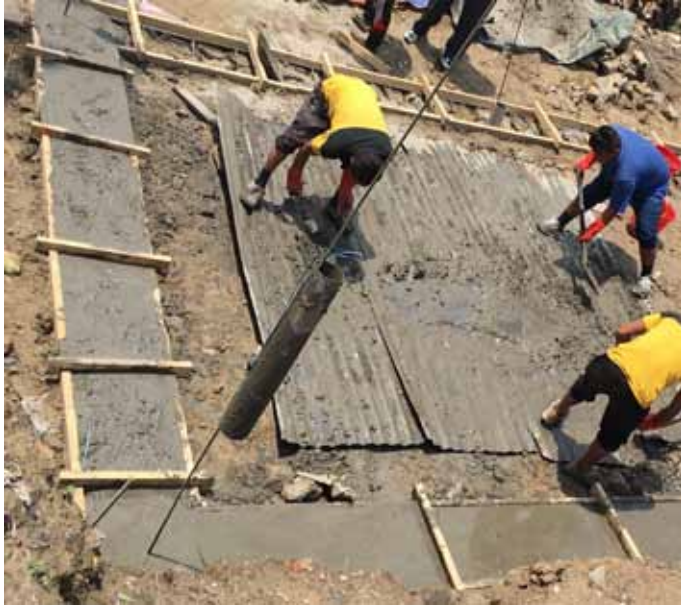
Then filling the rest of the band formwork
