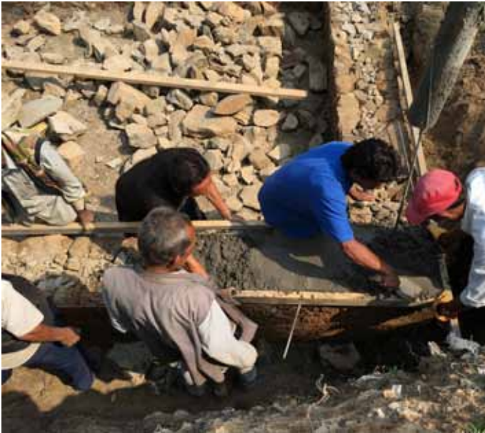
2' L band troweled on to 3" using sand and cement mortar mix
