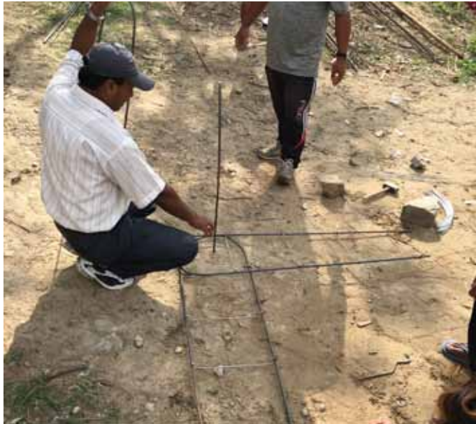
Bishnu explaining the different configurations of L and T bands
