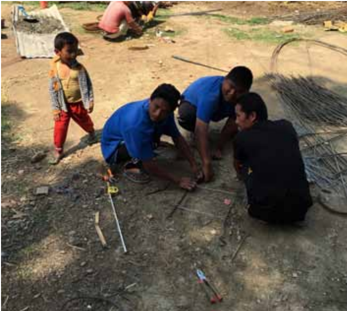
Securing the 3mm tie wires
