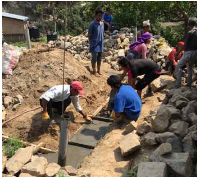
Then pouring of the band - 8 bags cement used to this point
