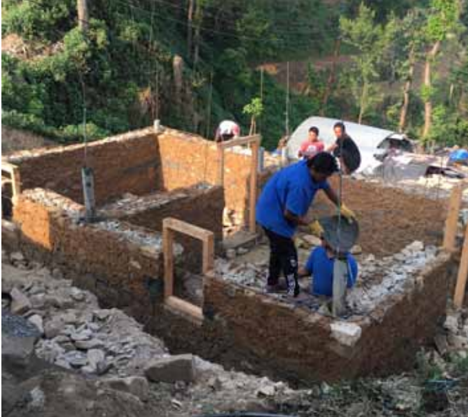
Gradual lifting of pipe as concrete is poured prevents it getting stuck
