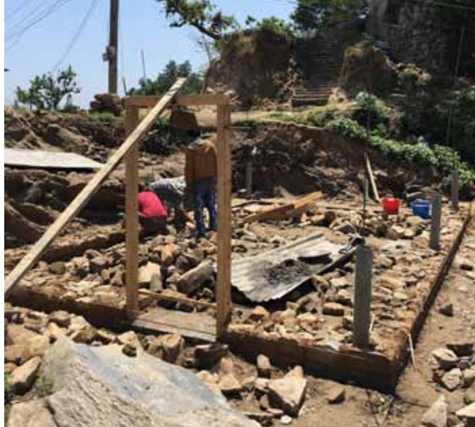
Door installed taking care to ensure 4' offset from any outside walls, allowing for L reinforcement
