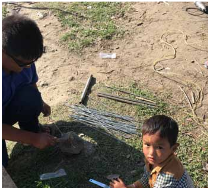
Cutting and straightening 3mm tie wire roll ready for use onsite
