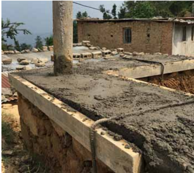
Banding team came up with a new way to hold formwork in place using bent steel bar
