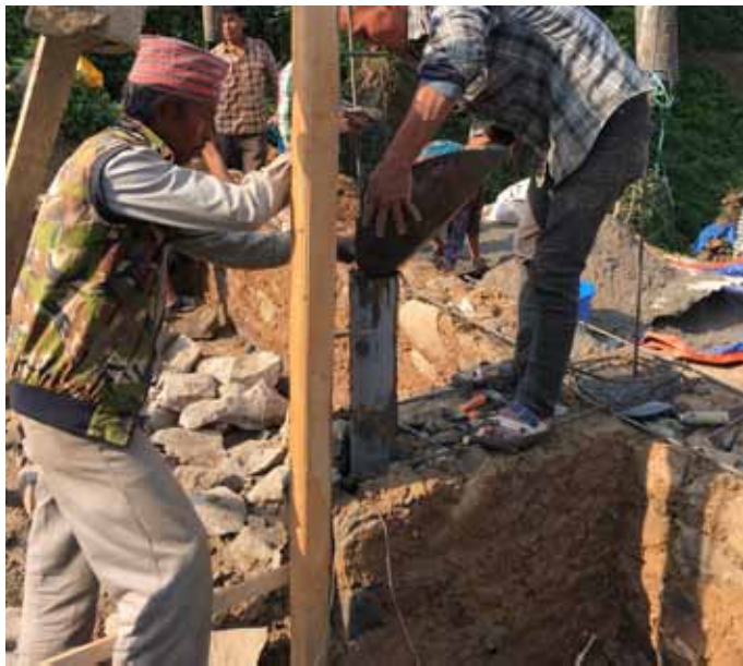
Core hole being poured, also "hold pass" concrete anchor to door jamb tie shown poured below...needs to be allowed for in materials
