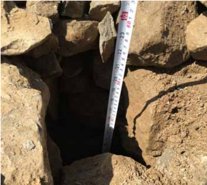
Checking depth is 2'
