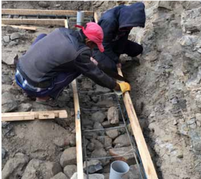
3mm wire ties to form steel reinforcement ladder
