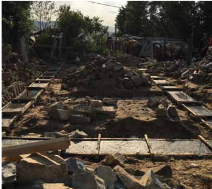
Completed band before clumps laid
