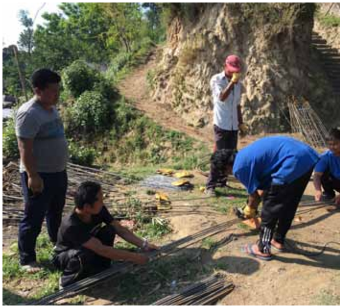
Cutting steel reinforcement for band no.1 at foundation level
