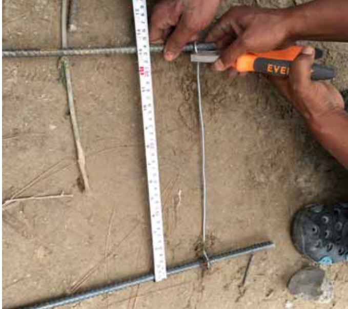
Secure the 3mm wire ties well around the steel bar to prevent it slipping out
