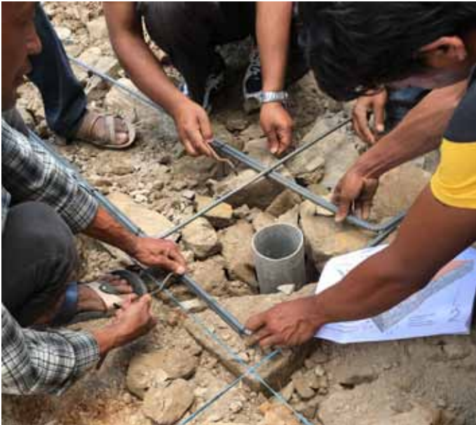
Bending 4' x 4' L rods connecting straight steel runs in first band
