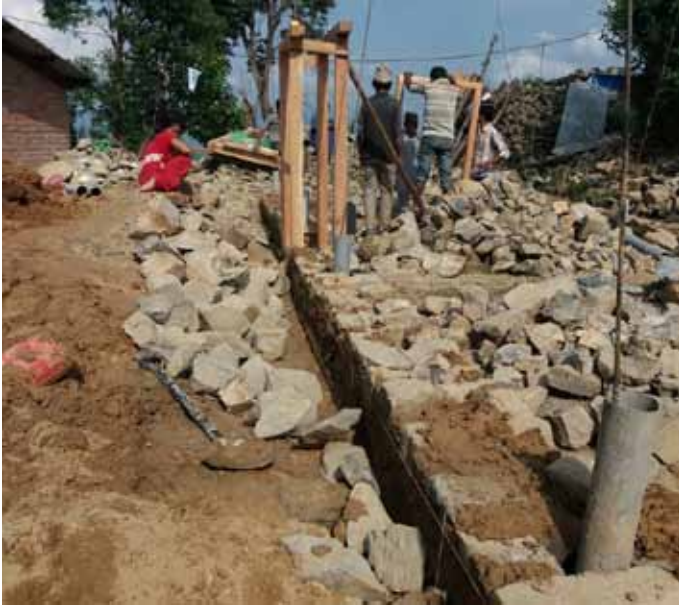
Doors being supplied and located in the plan by the householders
