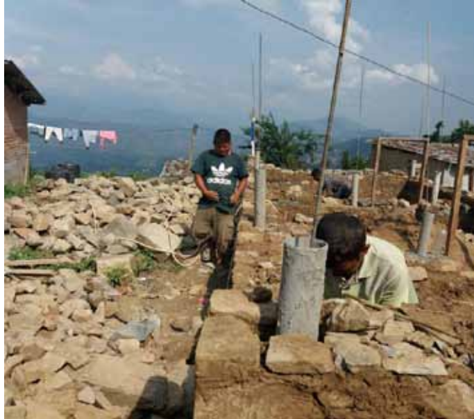
Stone masons progressing following completed 2' banding - photos this page by Surya Tamang the next week
