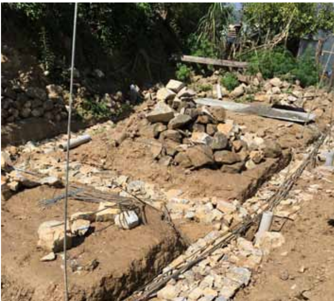
Stone laid into footing trenches, purchased by the household due to insufficient stone onsite
