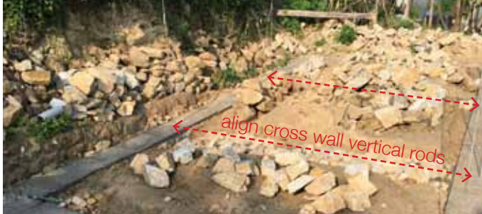
Check foundation trench depths and alignment of vertical rod core holes at cross walls
