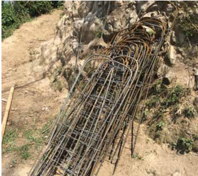
Prefabrication of steel elements in central location
