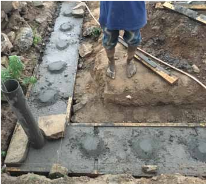
Clumps installed when it was realised time would not permit the masons from completing the first layer of stone before the concrete set
