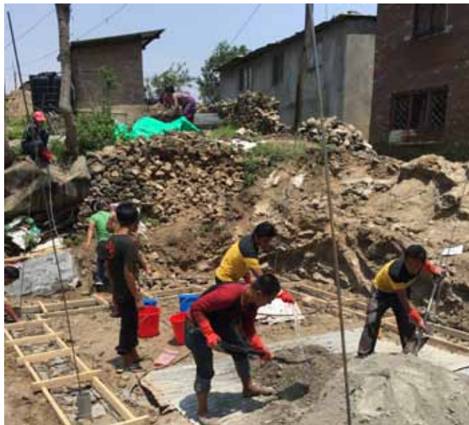
Concrete is batched onsite....
