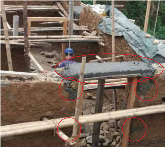
Add "hold passes" and window/door lintels to cement calculation
