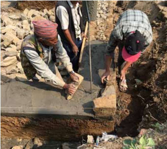
Stones being laid while mortar wet to maximise grab between stone and cement
