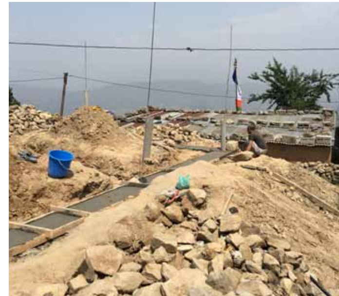
The completed foundation band with stone masons commencing laying of stone
