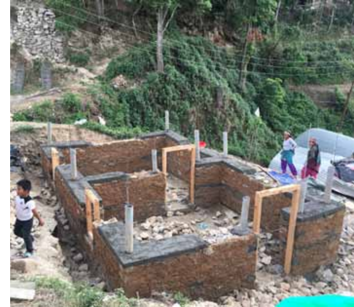
Completed L, T and cores...clumps to follow
