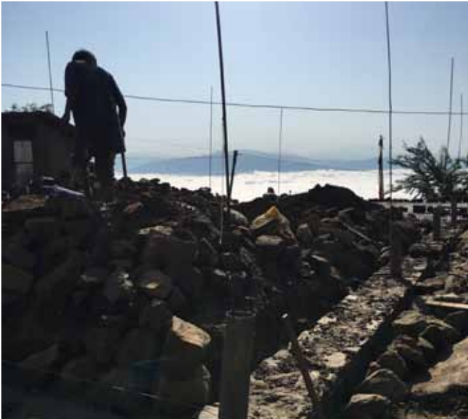
Mud from excavated footings being used to build the walls with minimal waste
