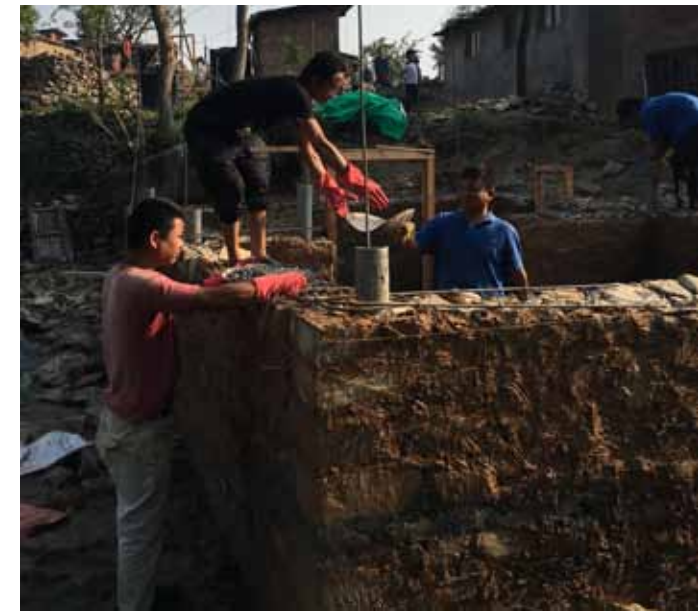
Concrete mix being poured into 4' band core holes
