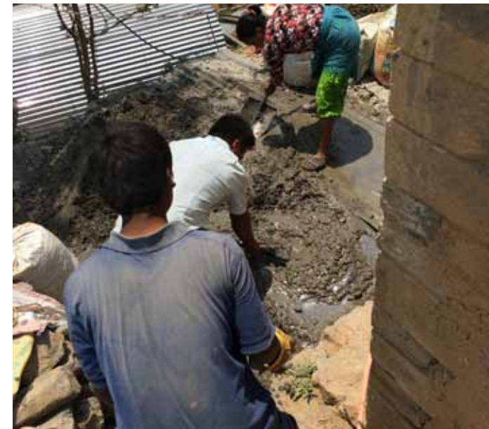
Manual batching of the cement by the householder
