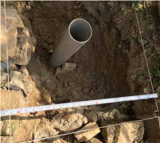
Household requested to dig down for vertical rod and footing depths and widths re-checked
