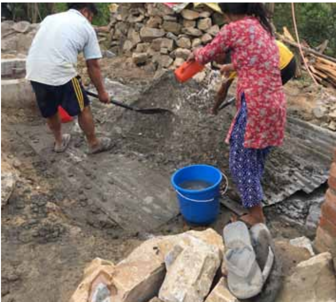
Batching concrete for band 1
