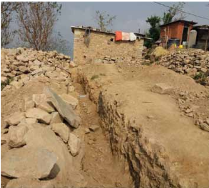
Trenches for foundations dug before arrival
