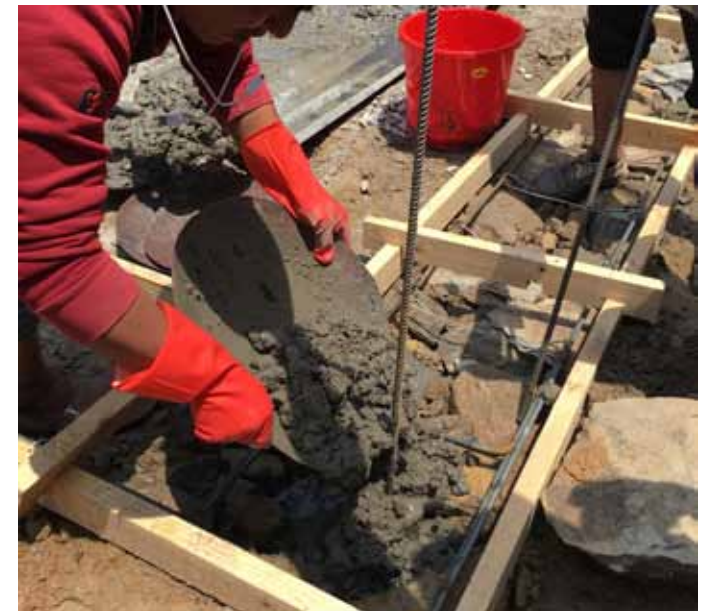
First placing concrete into the 4" core holes
