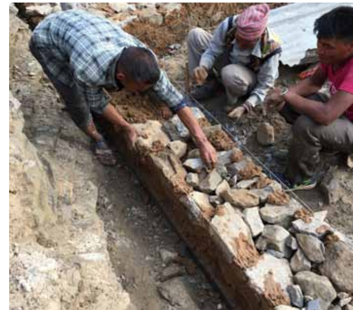
The stone mason team supplied by the householder laying the first two feet of wall
