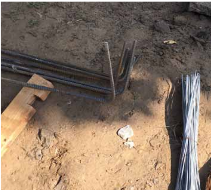
Cogs to bottom of verical rods tested on all sites and works welll, material efficient and is simple to work around
