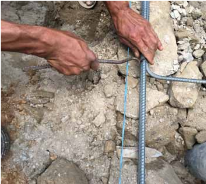
1mm wire ties to hold rods together
