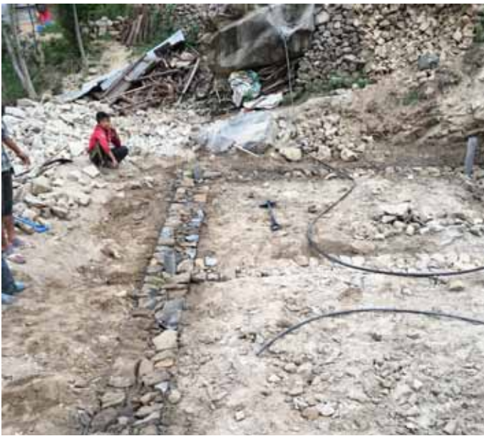
Stone laid into foundation trenches
