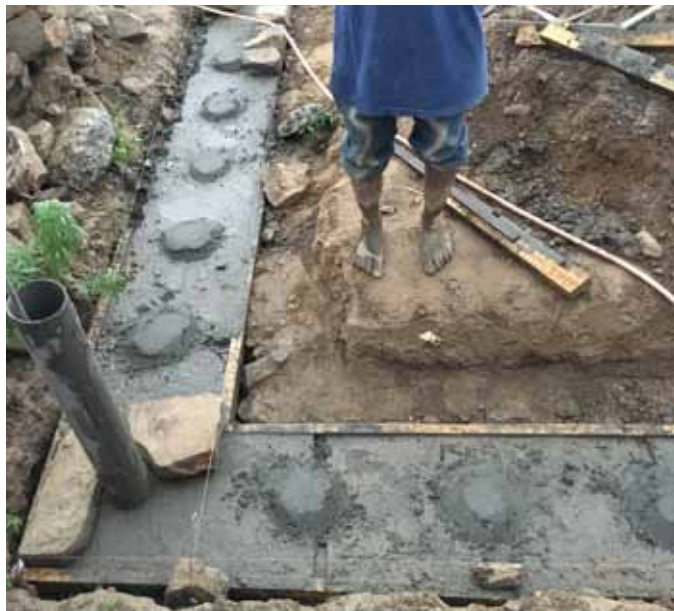
At H2 (Bambo) the clumps were poured while the band was wet, this is best practice
