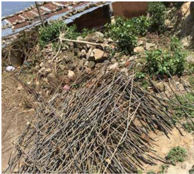
Pre-bent loops for all 3 house site prepared in one central place due to availability of space and power for the angle grinder
