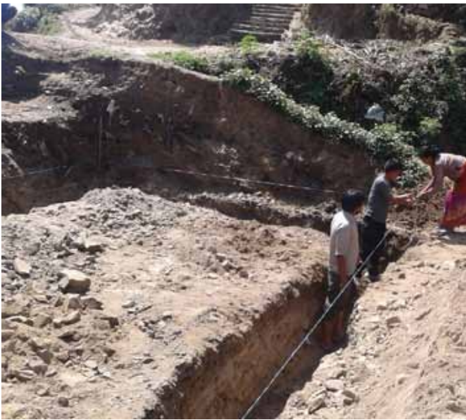
Foundation trenches being dug
