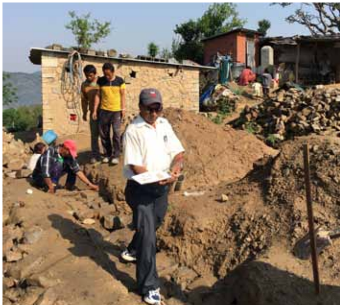
Checking trench and footing dimensions on arrival to site
