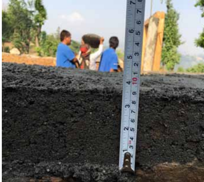
Avoid mortar bed depth exceeding 3" at T's and L's
