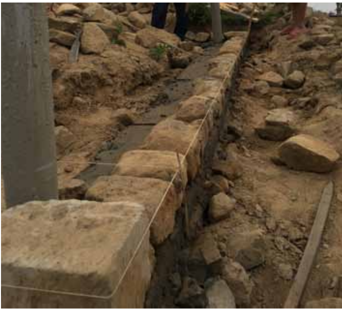
Stone being laid while the band is wet to maximise grab between stone and cement
