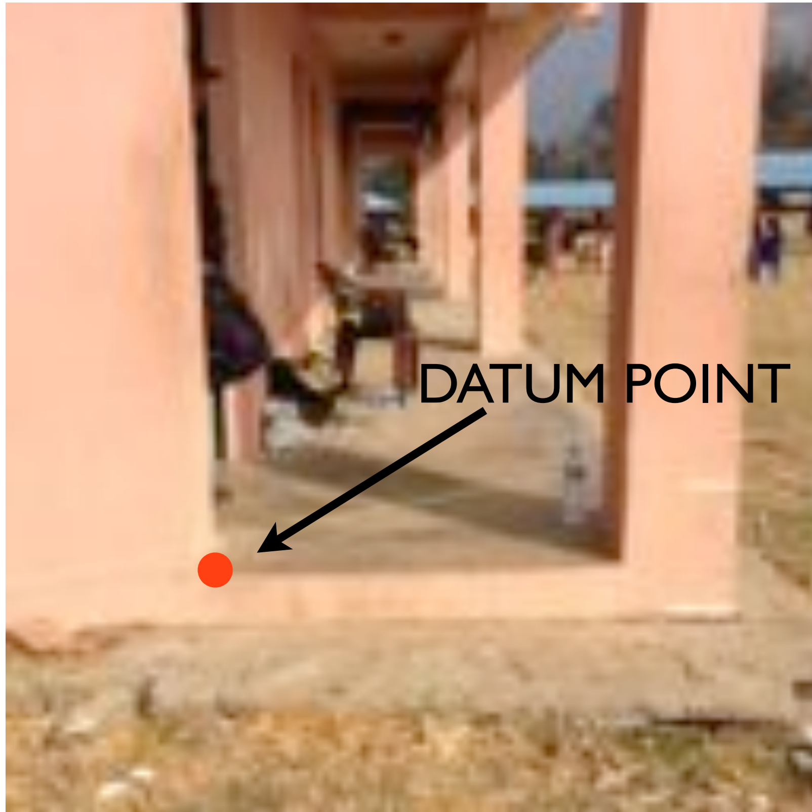
THANGPAL DHAP Setout datum for building work Finished floor level (FFL), edge of slab, corner of building
