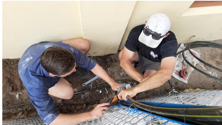
The water line into the tank and from tank to the hand washing and to the toilets.
