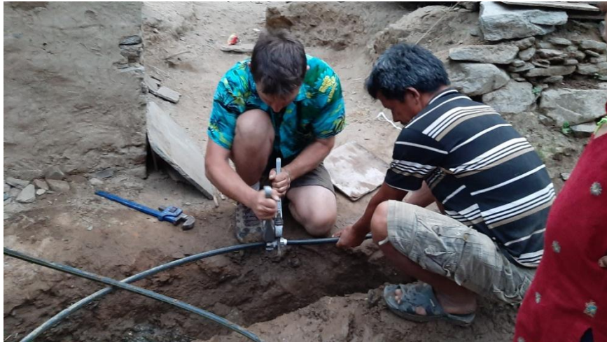
The damaged water line was reconnected.
