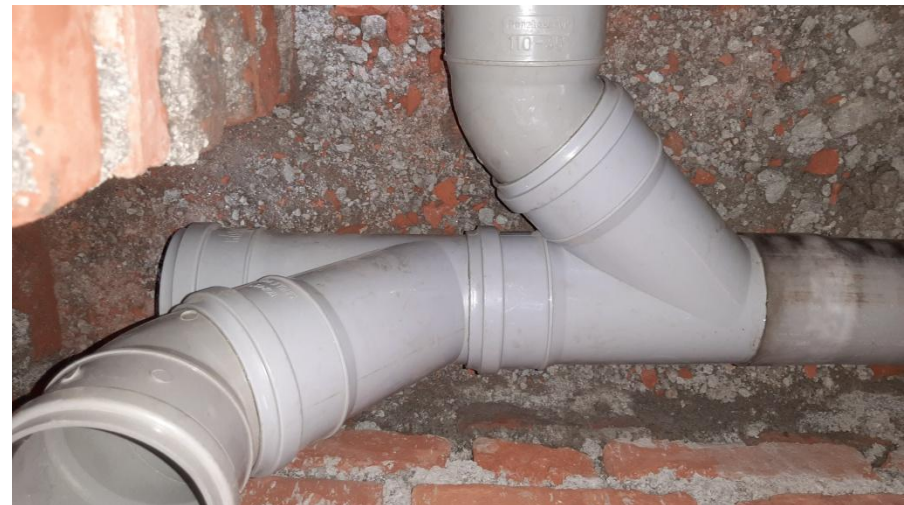
Hand washing waste pipe line fitting at Saraswoti Basic School, Lapse.
