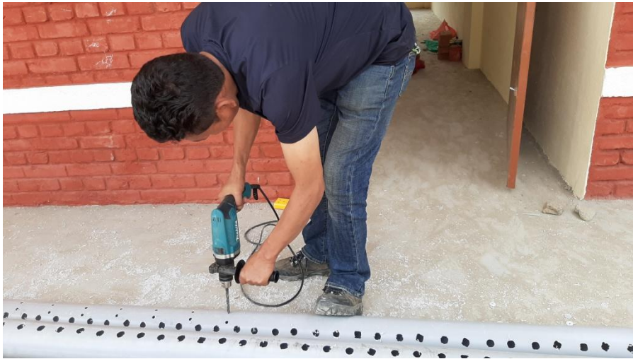
Soakage trench pipe preparation
