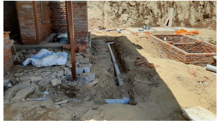
Drainage from hand washing taken to septic system.
