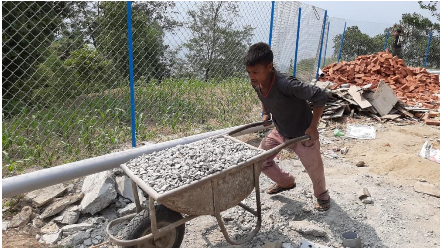
The Soakage trench pipe covered with gravel.
