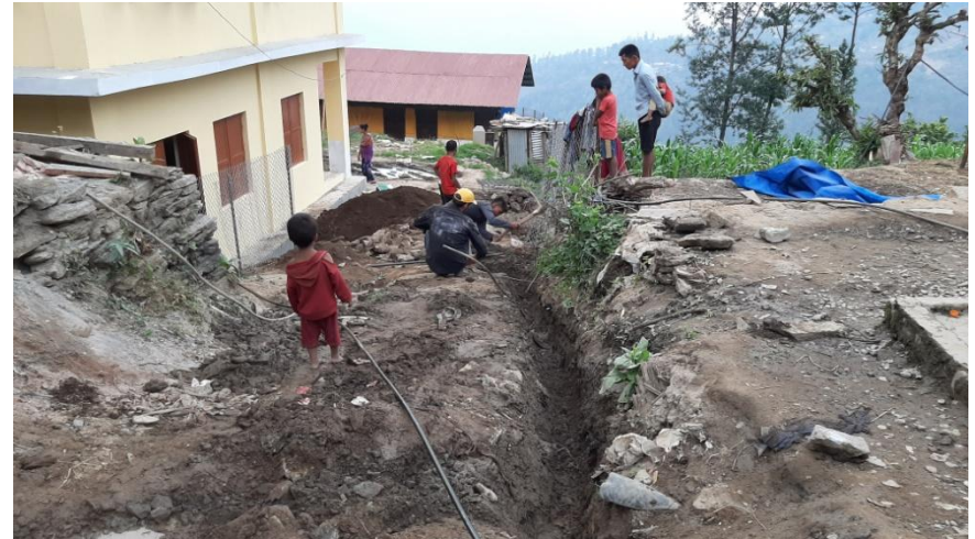
The poly pipe water line was taken to the school beside the road to the school.
