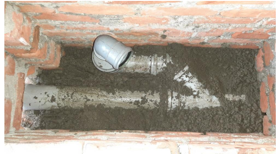
Hand washing area drain pipe work...
