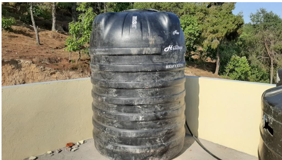
Water tank of 2000lit capacity installed at Panchakanya School.
