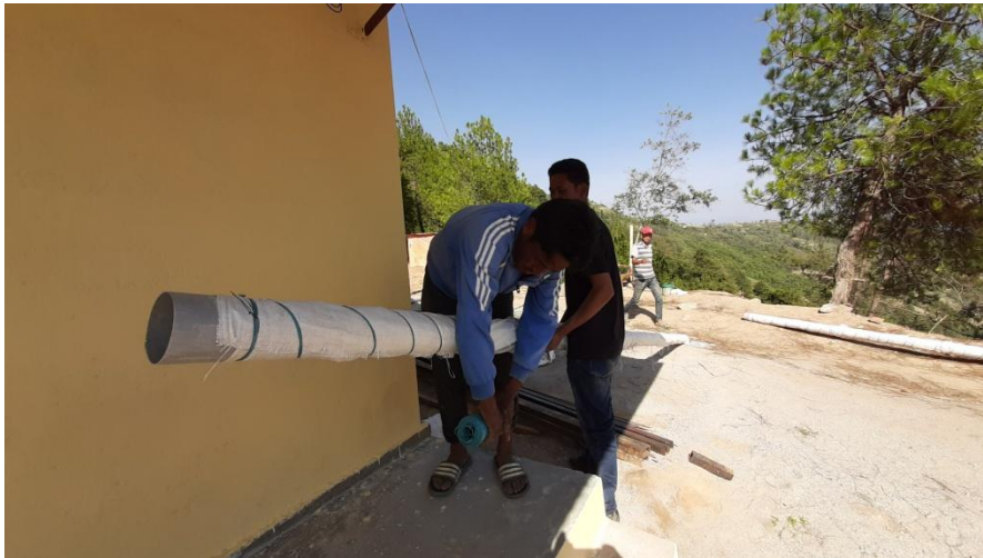
Cement bags wrapping on to Perforated Soakage trench pipe
