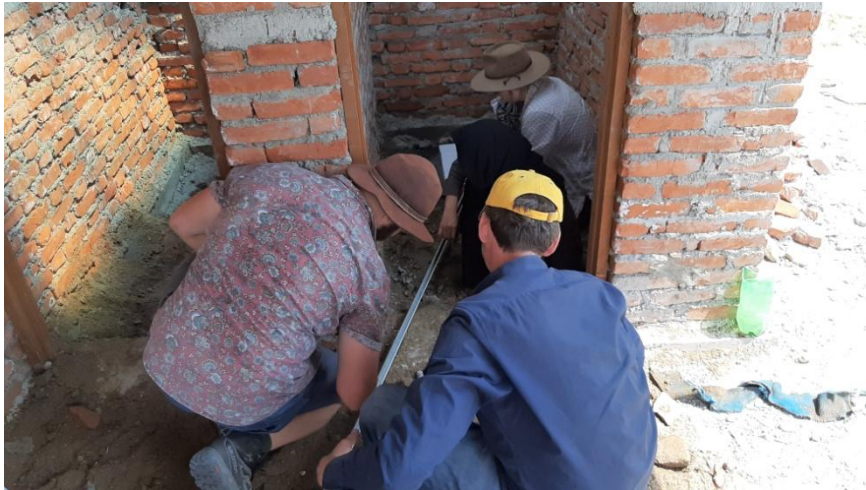
Checking of floor level down fall to toilet pan
