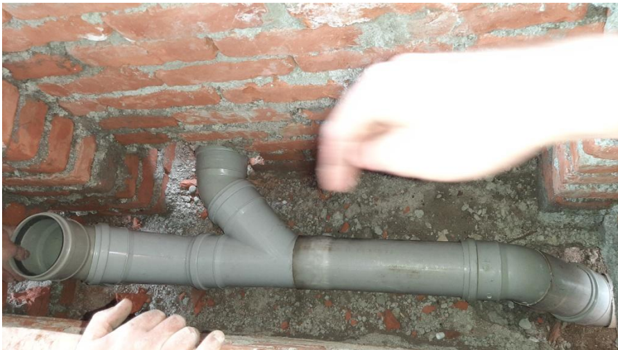
Hand washing waste pipe line fitting at Saraswoti Basic School, Lapse.
