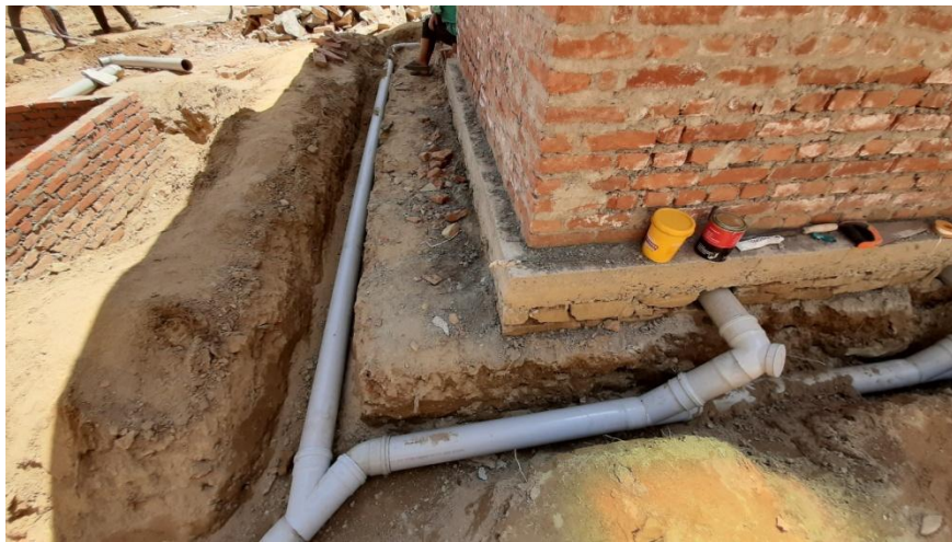
Y- Tee Junction drainage connection for toilet and hand washing
