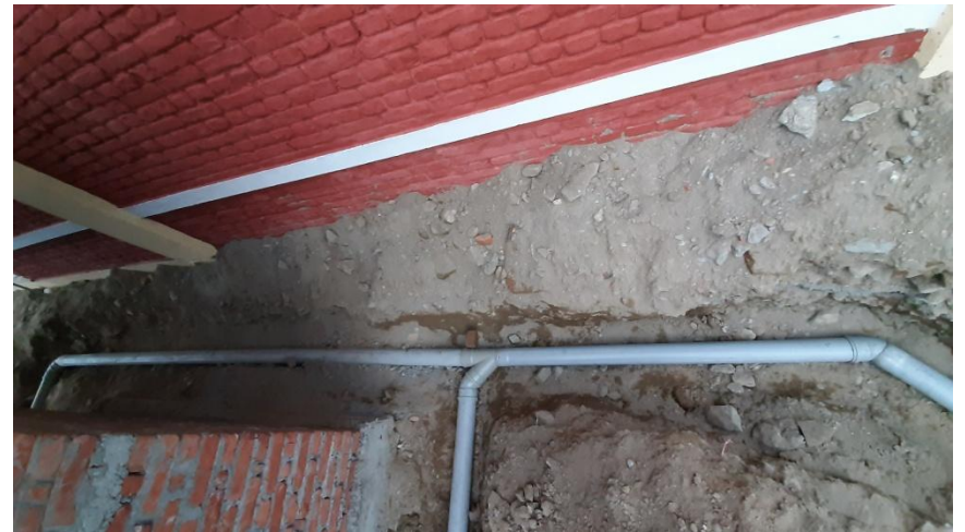
Drainage line from toilet and hand washing taps taken into the septic tank.
