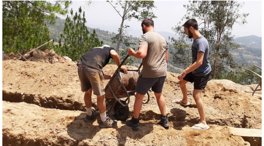
The studio team assisting in covering the soakage trench pipe at panchakanya school
