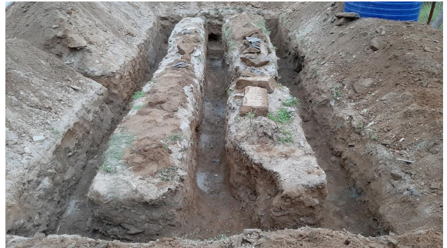
Soil excavated Soakage trench
