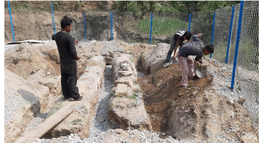
The Soakage trench was covered by soil as the top layer of the trench.
