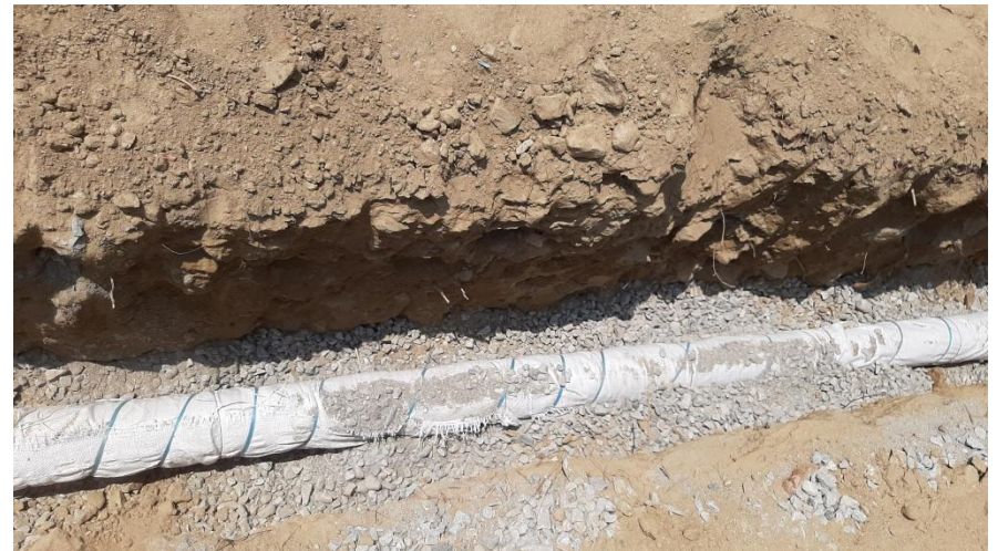
Soakage trench pipe laid and covering with gravel
