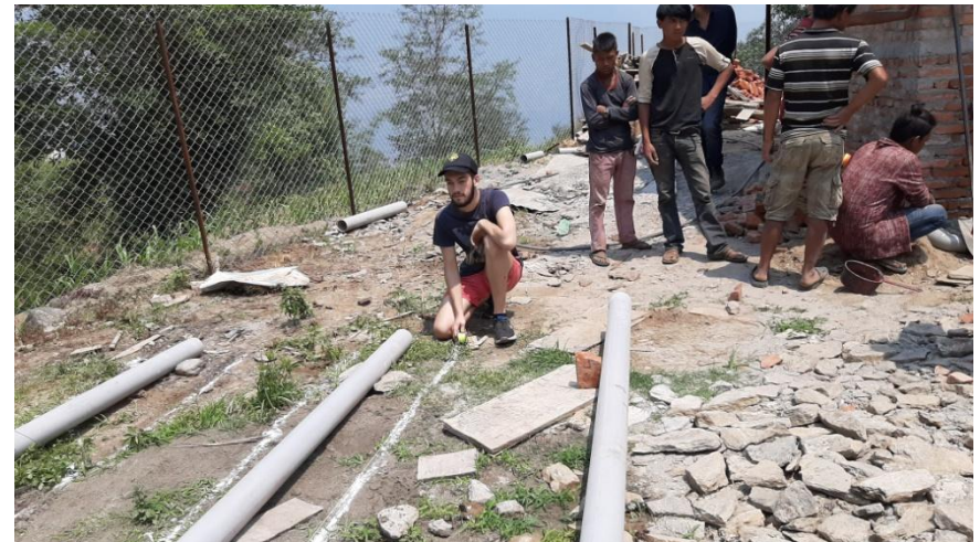
Soakage trench marking for soil excavation
