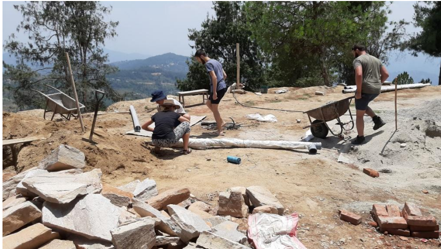
The studio team assisting in covering the soakage trench pipe at panchakanya school
