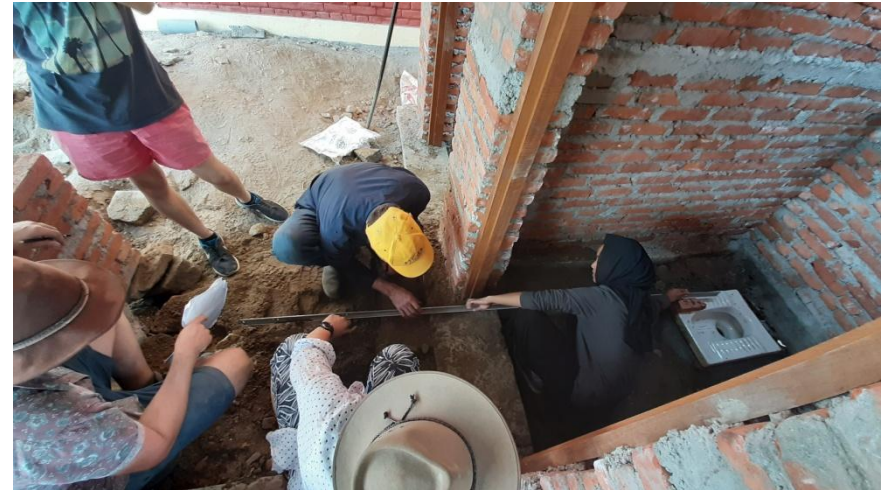
Checking of floor level down fall to toilet pan
