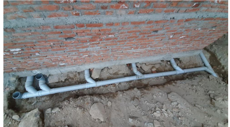
Toilet drainage with Inspection Opening and Vent Pipe placement setting at Saraswoti School.
