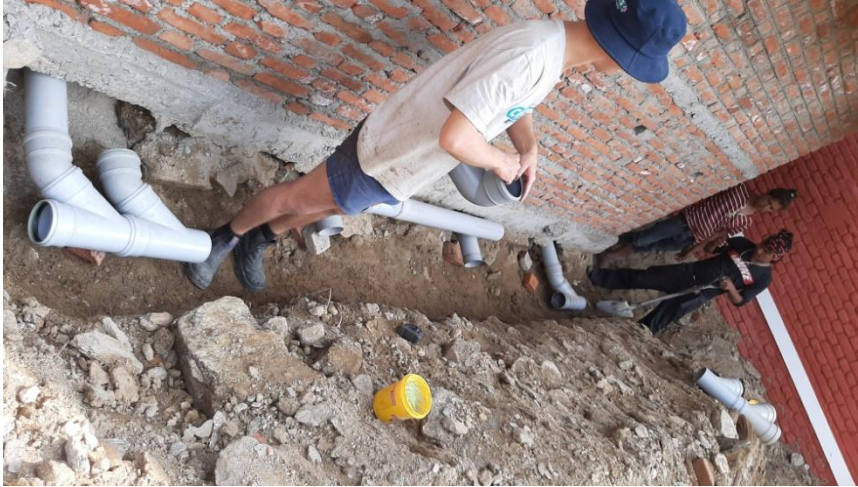
Setting up of toilet drainage
