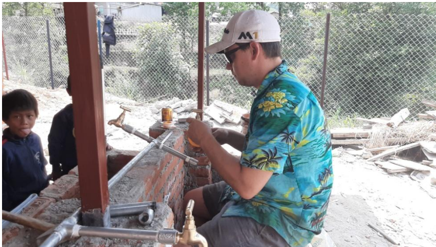
The water work – Taps for drinking water and hand washing at Saraswoti School, Lapse.
