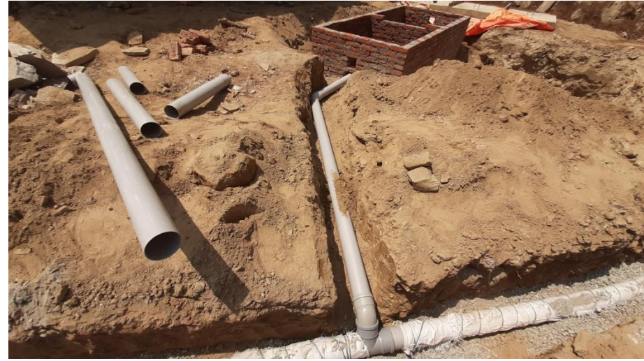
The drainage work – connections from septic tank to Soakage trench.
