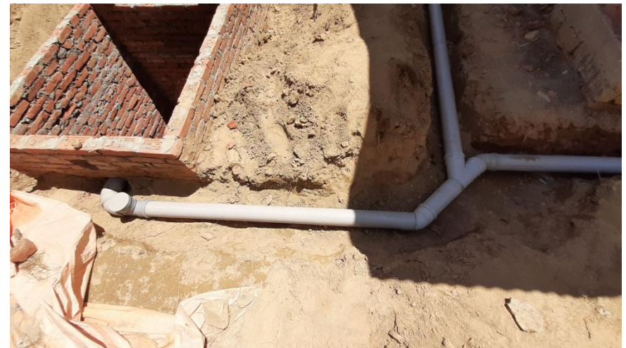
Y- Tee Junction drainage connection of toilet and hand washing joined in to the septic tank.
