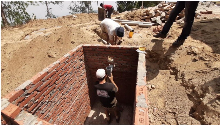
The drainage work – connections from septic tank to Soakage trench.
