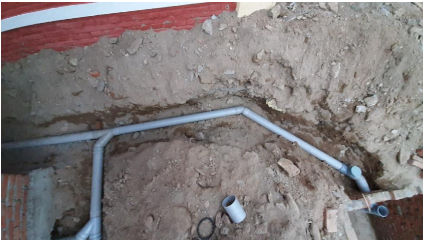
Drainage line from toilet and hand washing taps taken into the septic tank.
