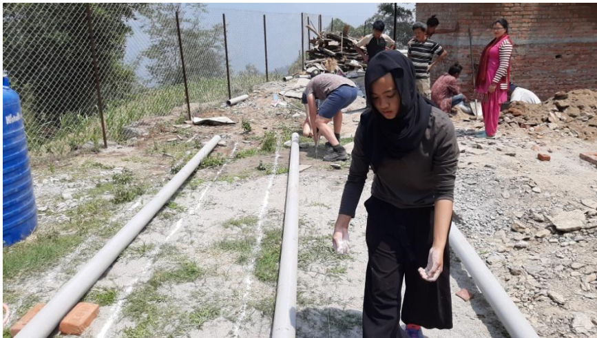
Soakage trench marking for soil excavation
