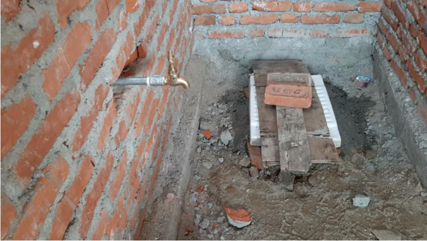
Water line and tap placed inside the toilet.
