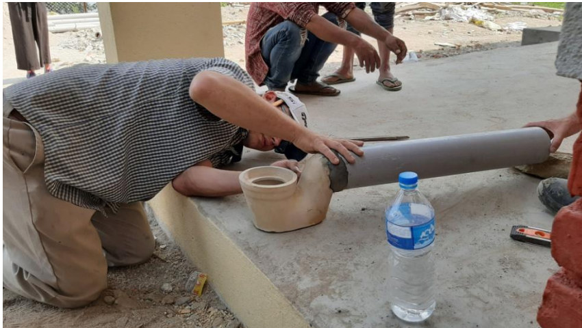
PVC outlet pipe setting to CYPHON of the Asian style toilet pan.
