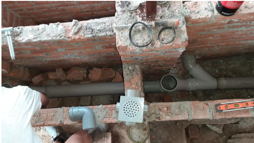
Hand washing area drain pipe work...
