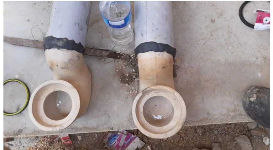
PVC outlet pipe setting to CYPHON of the Asian style toilet pan.
