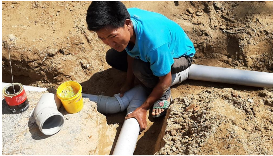
The drainage work at Panchakanya Basic School, Chamkhu, Jyamire.
