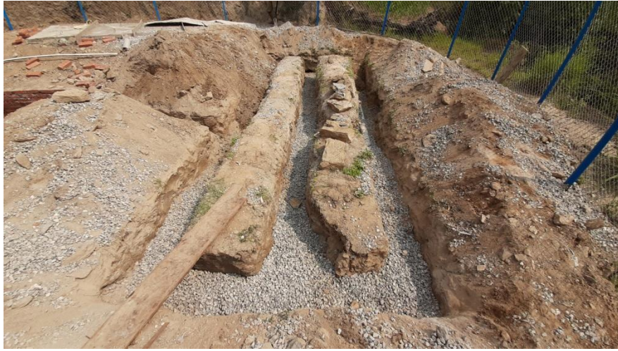
Soakage trench filled with gravel at bottom of the trench.
