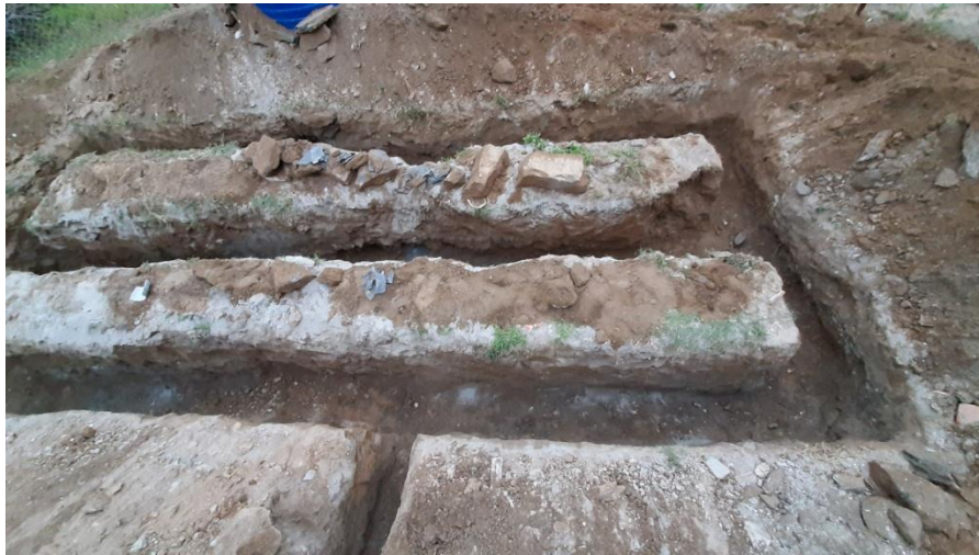
Soil excavated Soakage trench
