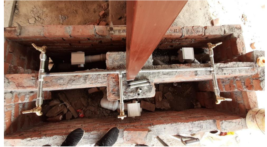
The water work – Taps for drinking water and hand washing at Saraswoti School, Lapse.
