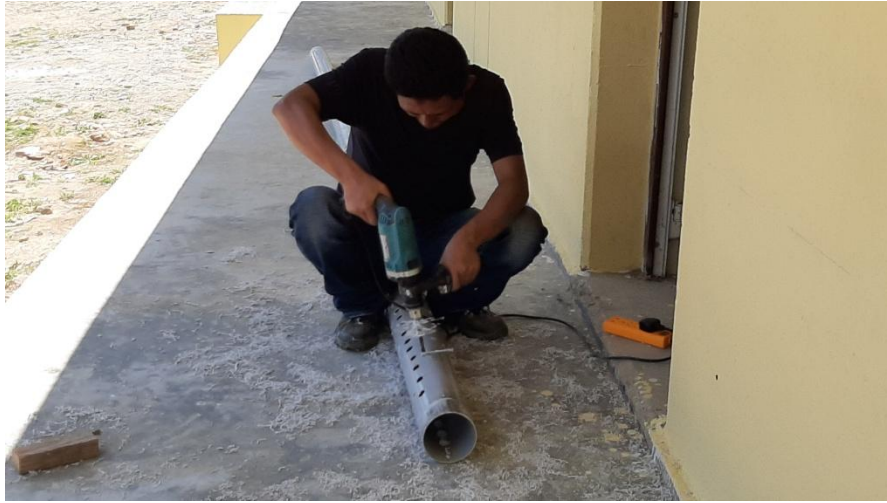
Perforating Soakage trench pipe
