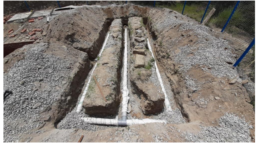
The Soakage trench pipe wrapped with cement bags laid into the trench.
