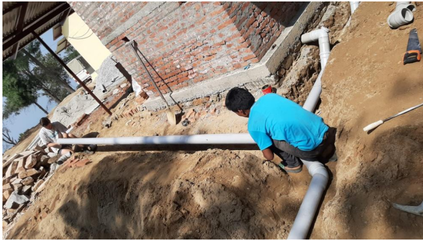
Drainage from hand washing taken to septic system.
