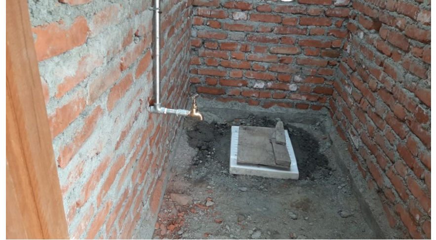
Water line and tap placed inside the toilet.
