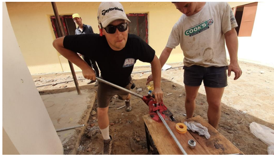
Making GI connections.
