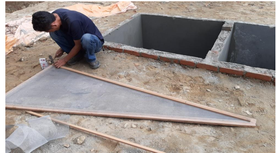
The stainless steel fly mesh securing by adding piece of timber on top of fly mesh.
