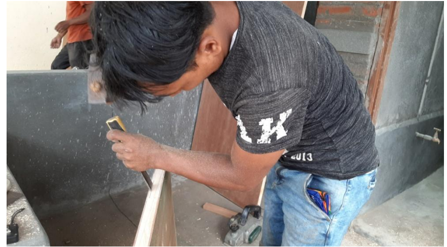
Prepararing for door hinges at Panchakanya Basic School
