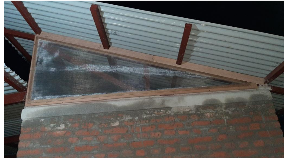
Fitting of the side way fly mesh at Panchakanya Basic school.
