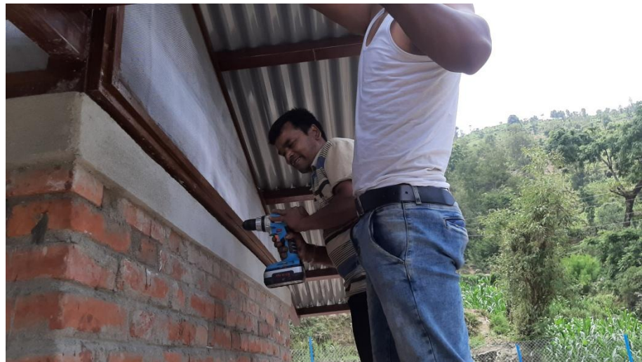
Fitting of side fly mesh at the side ventilations of the toilet block.
