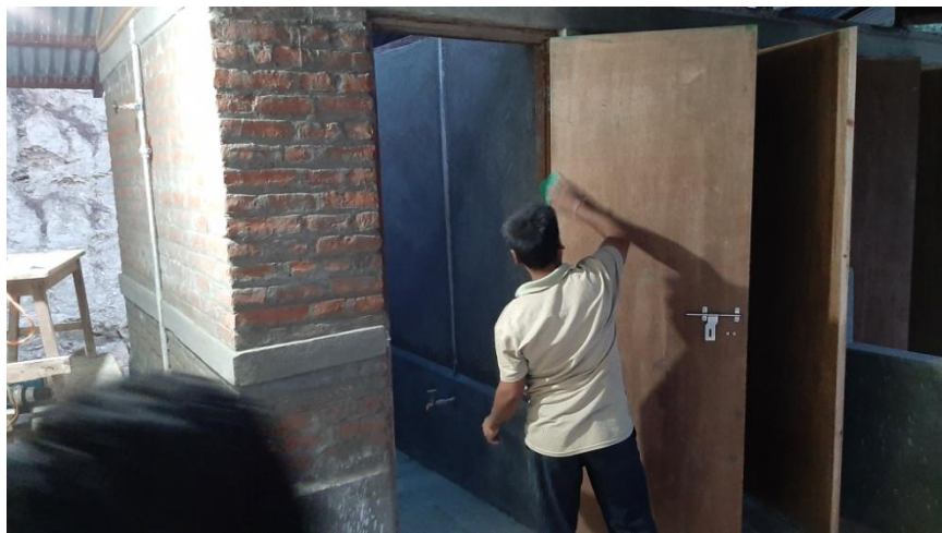
Cleaning of door with sandpaper prior to coloring on the door.
