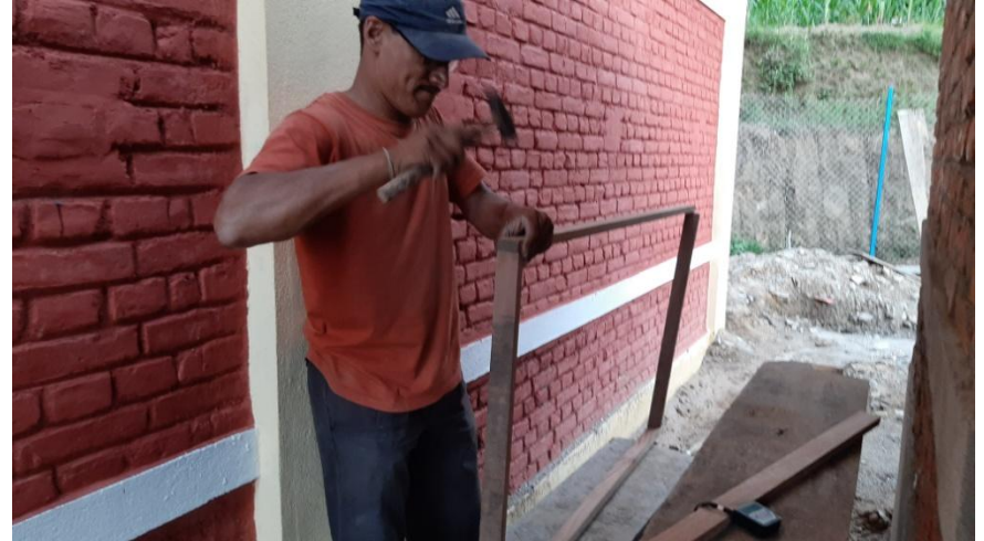
The front fly mesh timber frame preparation.
