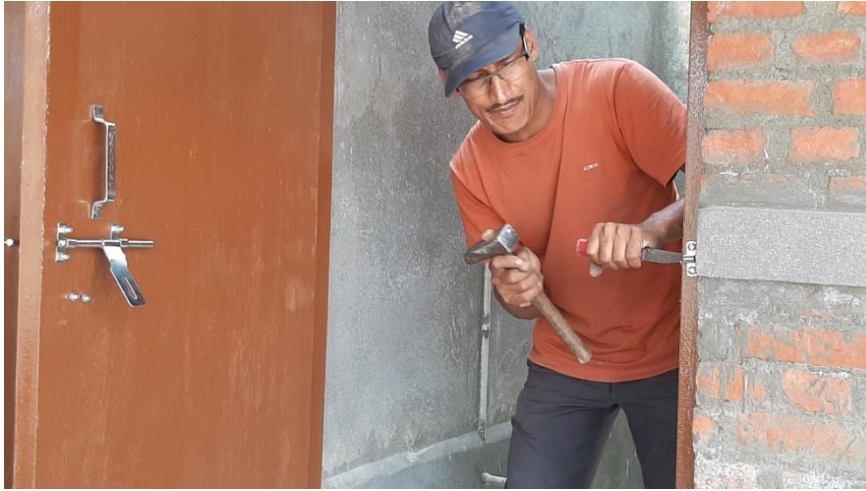
Making a smooth hole for the inside lock
