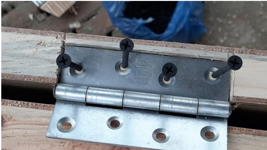
Hinges placing on the door prior to insert on to door frame.
