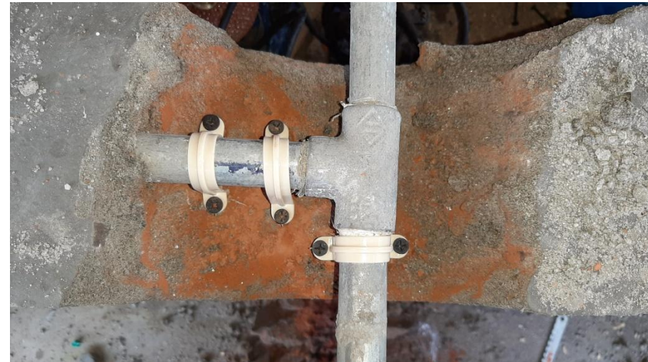
The clamps to secure hand washing tap pipes from getting loose.
