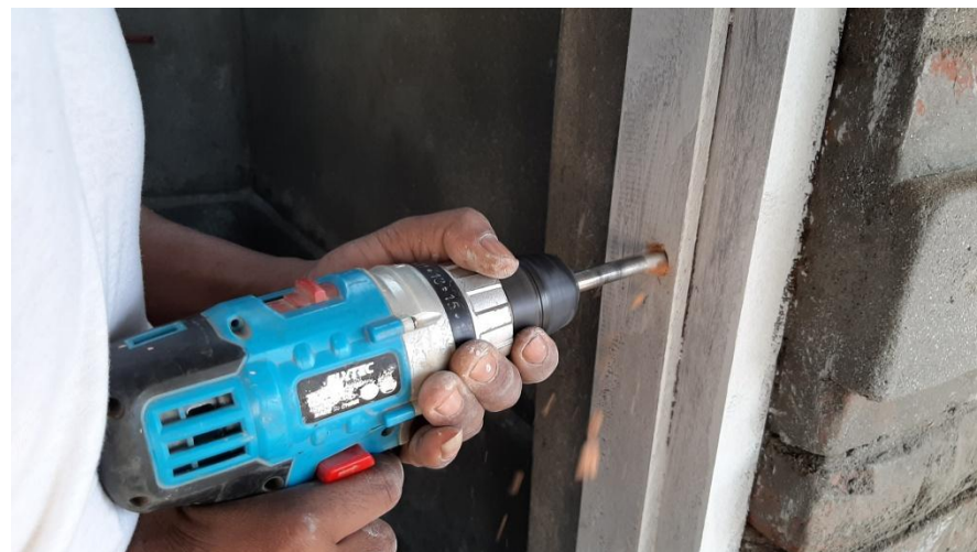
Making hole on door frame for inside door lock.
