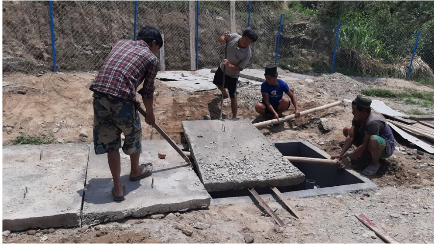
The septic tank was covered by prepared septic slab after removing all the water and stones/ brick pieces from the tank and sealed from top by joining the slabs with cement mortar at Saraswoti Basic School, Lapse.
