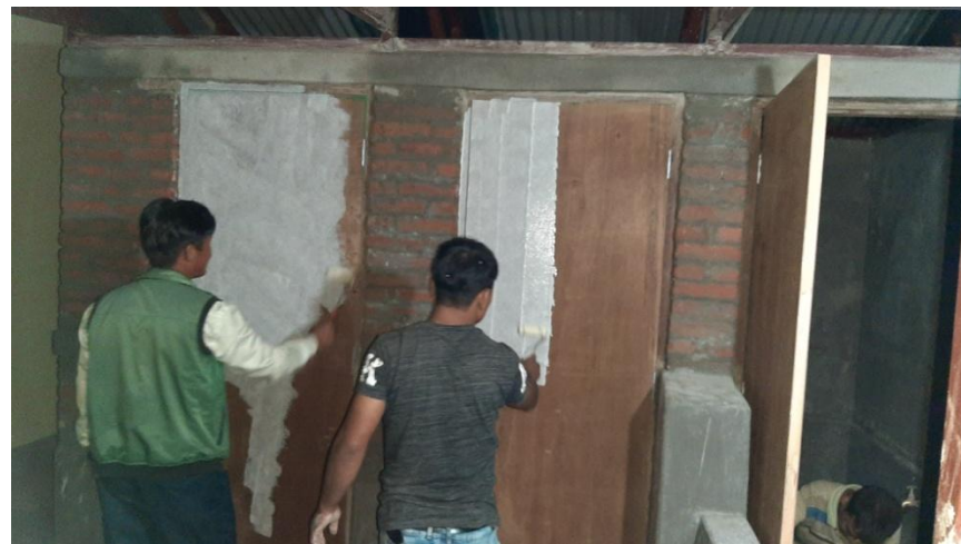
Wood Primer application prior to enamel paint.
