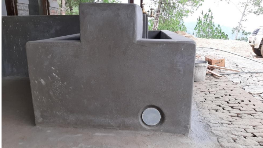
The Inspection opening for the tap
