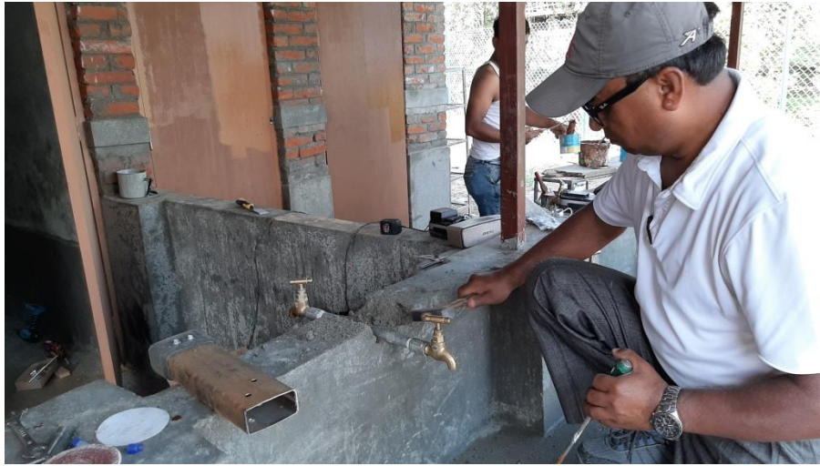
Breaking of render and hard render of the hand washing taps.
