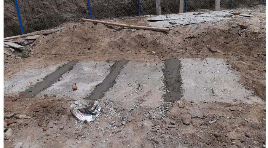
The septic tank was covered by prepared septic slab after removing all the water and stones/ brick pieces from the tank and sealed from top by joining the slabs with cement mortar at Saraswoti Basic School, Lapse.
