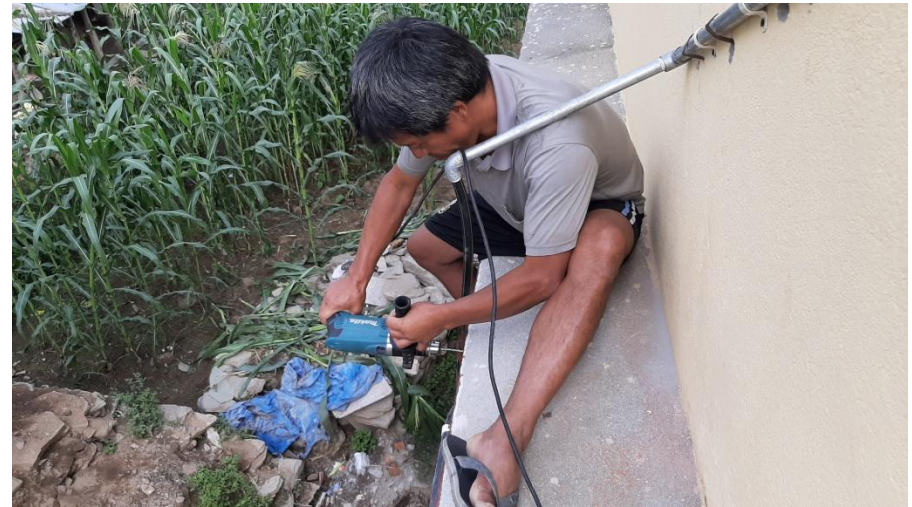
Securing the water pipes to water tank and from water tank.
