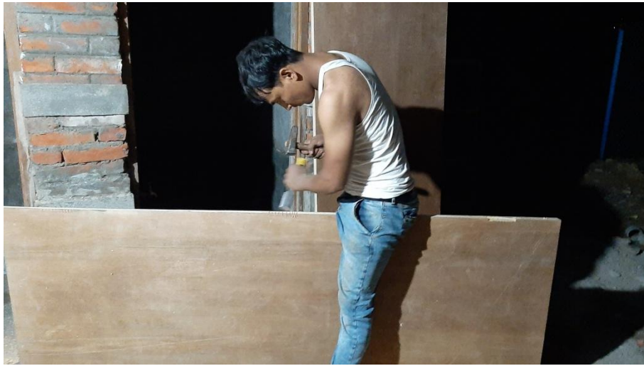
Setting of doors, placing door hinges
