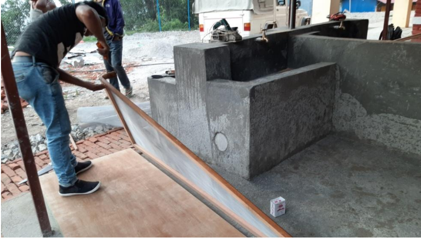
Preparation of side way fly mesh for side ventilation at Saraswoti School.
