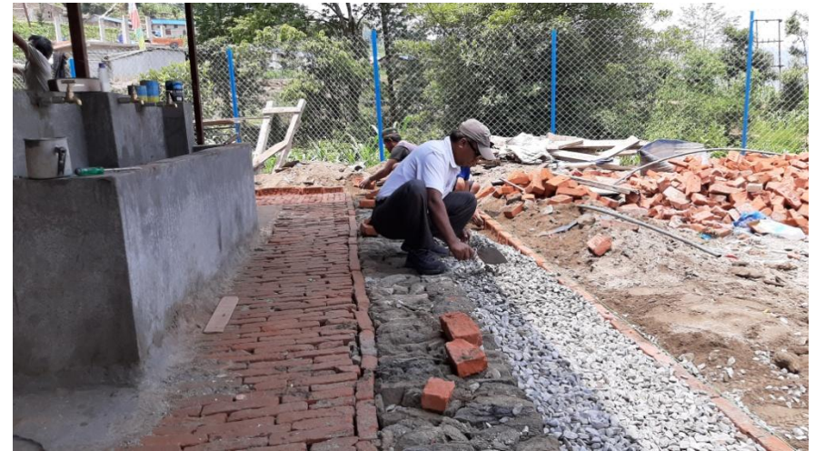
Stone soling after the brick soling around main front yard of the toilet block.
