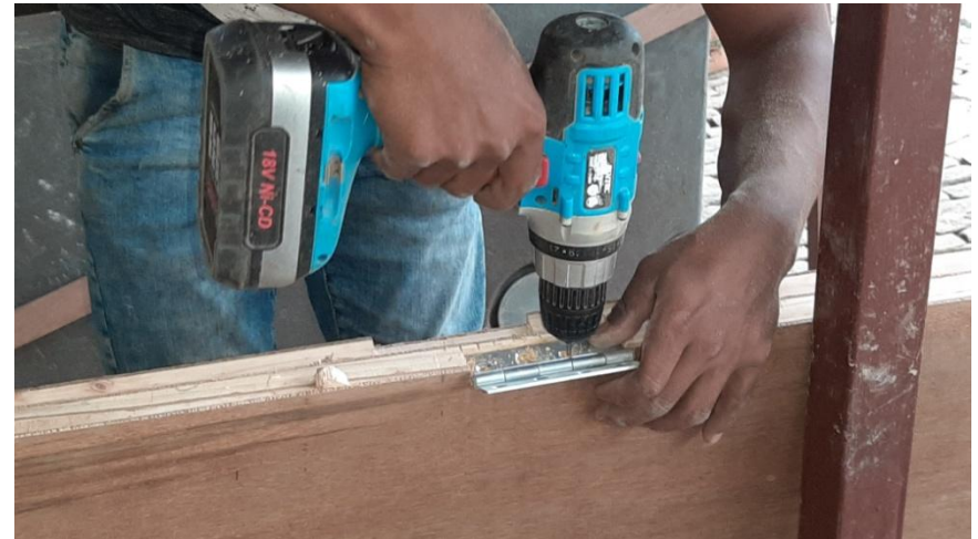
Hinges placing on the door prior to insert on to door frame.
