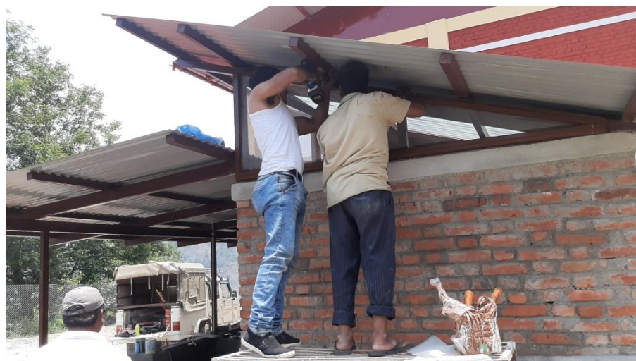
Fitting of side fly mesh at the side ventilations of the toilet block.
