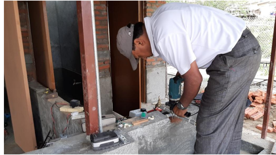
Breaking of render and hard render of the hand washing taps.
