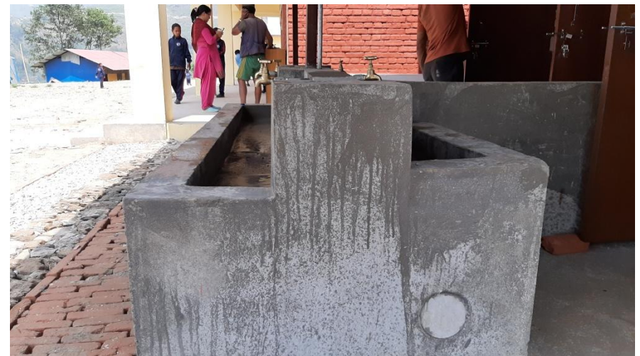
The Inspection opening for the hand washing taps.
