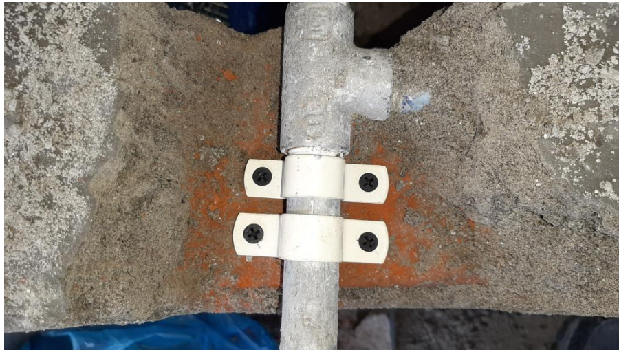
The clamps to secure hand washing tap pipes from getting loose.
