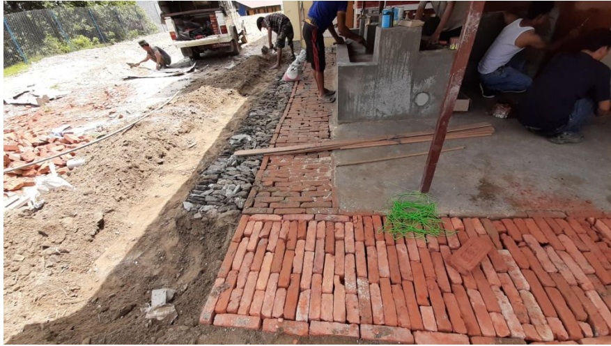
Brick soling around main front yard of the toilet block.
