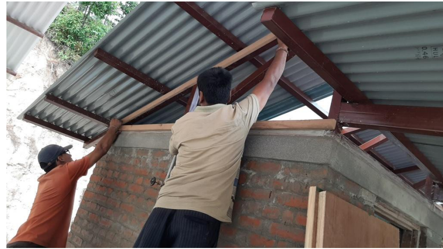
Measuring of the timber pieces to make side ways fly mesh frame
