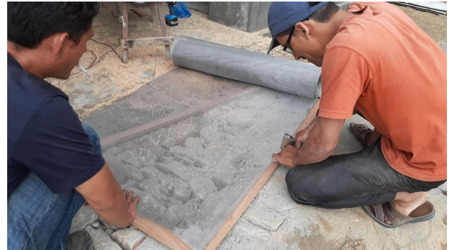
Applying the fly mesh on to the fly mesh timber frame.
