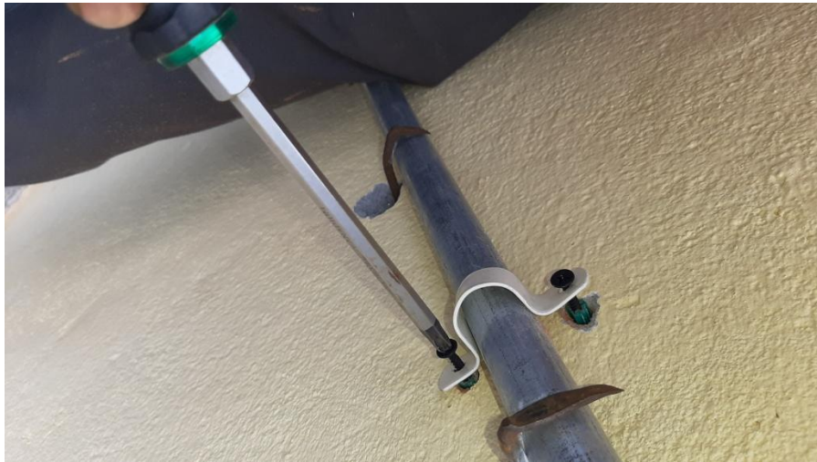
Securing the water pipes to water tank and from water tank.
