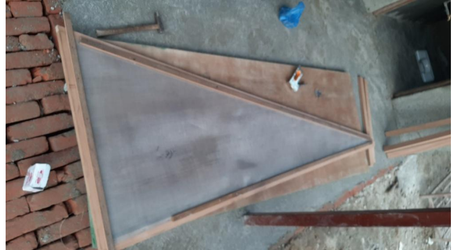
Preparation of side way fly mesh for side ventilation at Saraswoti School.
