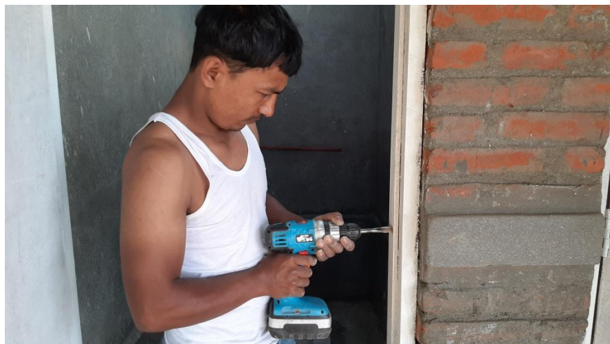
Making hole on door frame for inside door lock.
