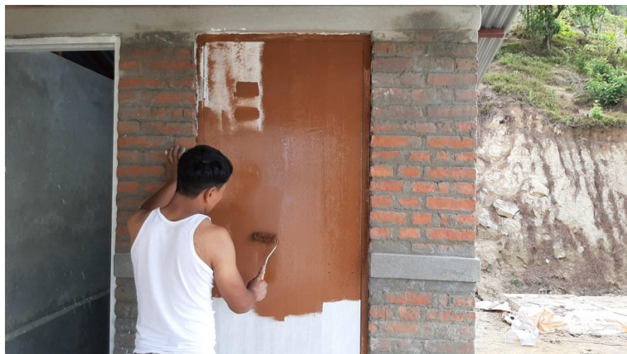
Door painting with enamel after wood primer was set dry..
