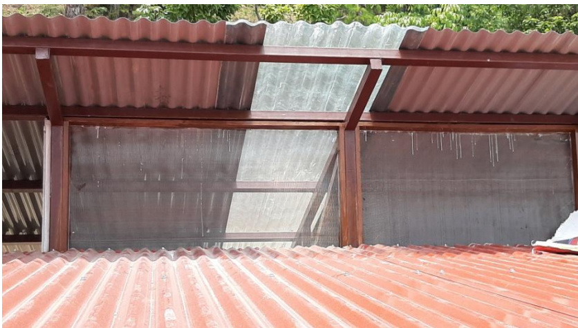
The front ventilation fly mesh work and coloring at Panchakanya Basic School.
