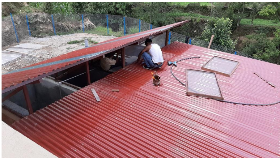
Fitting of the front fly mesh at the front ventilation of the toilet block.
