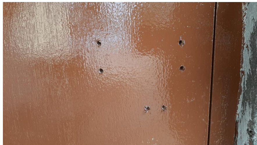
The enamel painted door with the hole created to insert outside and inside door latch.
