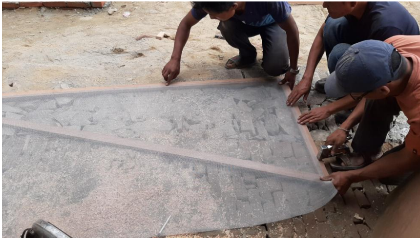
Applying the fly mesh on to the fly mesh timber frame.
