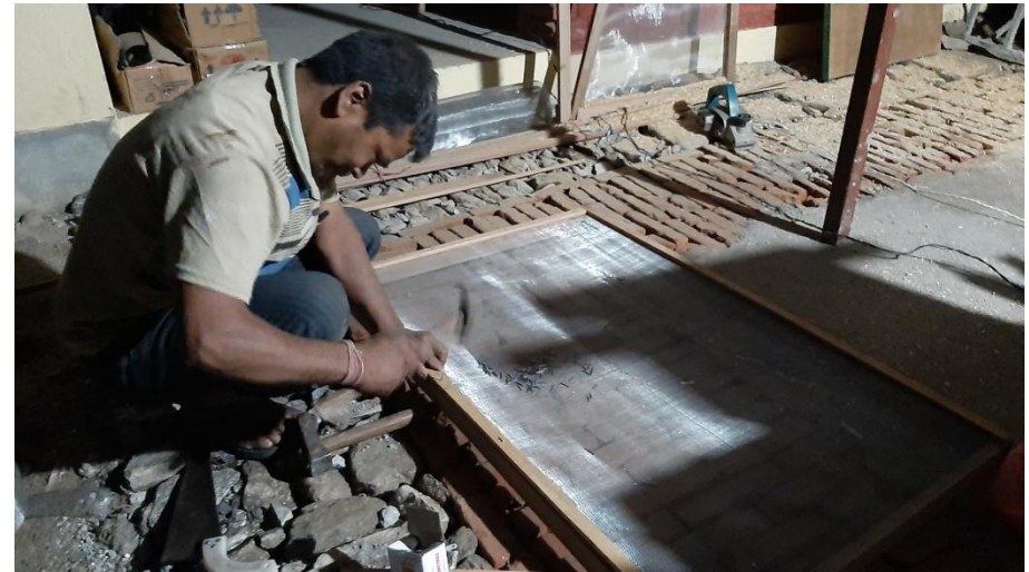
Setting of front ventilation fly mesh.
