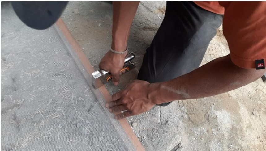
Stitching the fly mesh on to the fly mesh timber frame.
