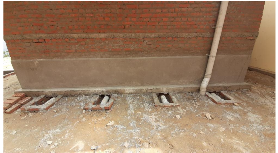
The toilet IO opening securing – The team will put an stone slate onto o f the brick walls.
