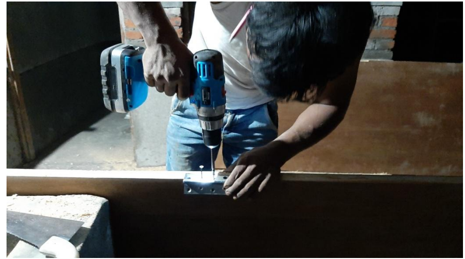
Setting of doors, placing door hinges
