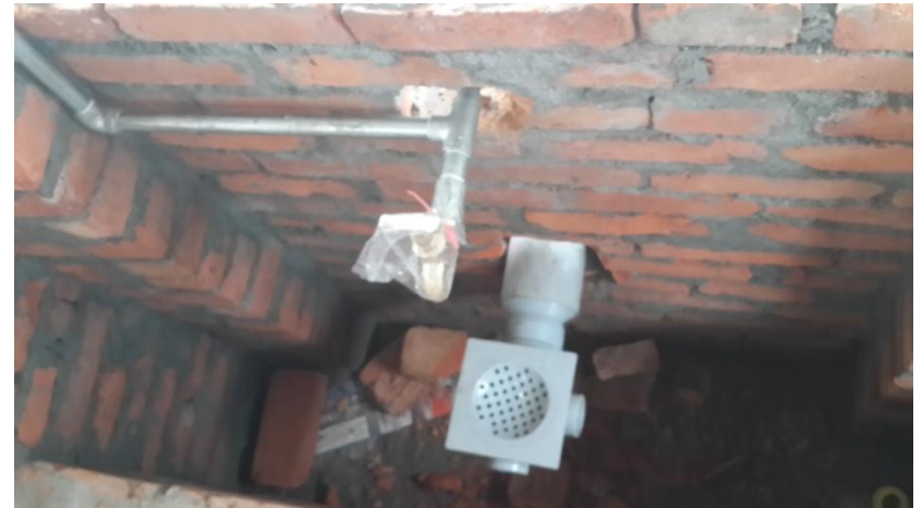
Drainage work for hand washing and water drinking taps.
