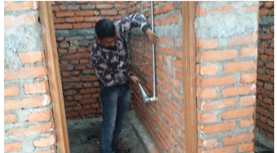
Vilas Dian working to install taps inside the toilet
