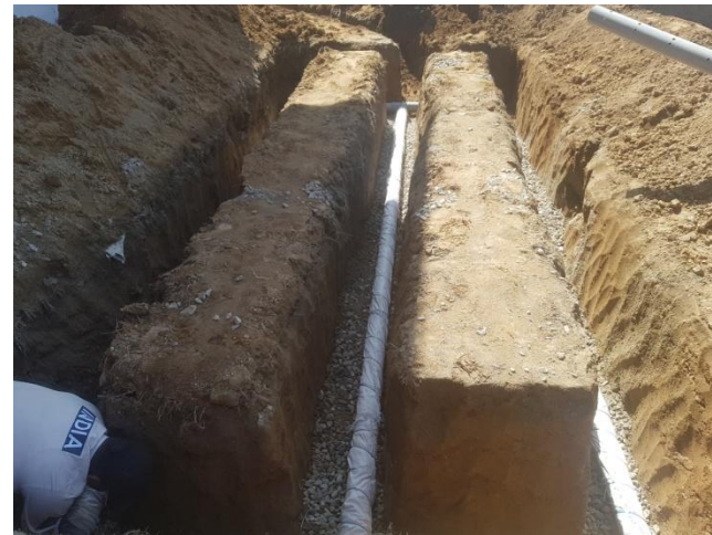
Placement of perforated cement bag wrapped pvc pipe
