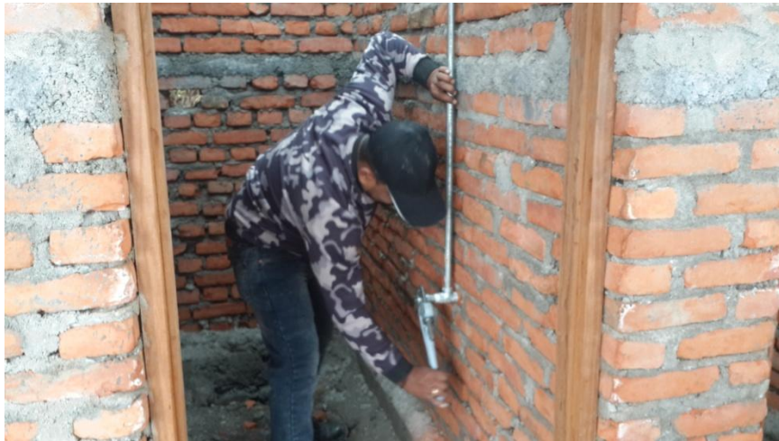
Vilas Dian working to install taps inside the toilet
