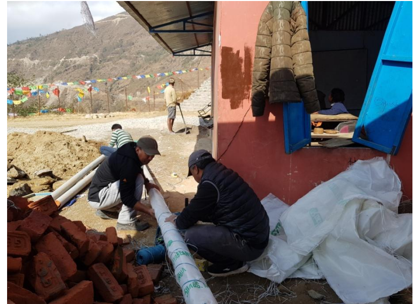
Wrapping of the perforated PVC pipe by CEMENT BAGS before laying onto the soakage trench..
