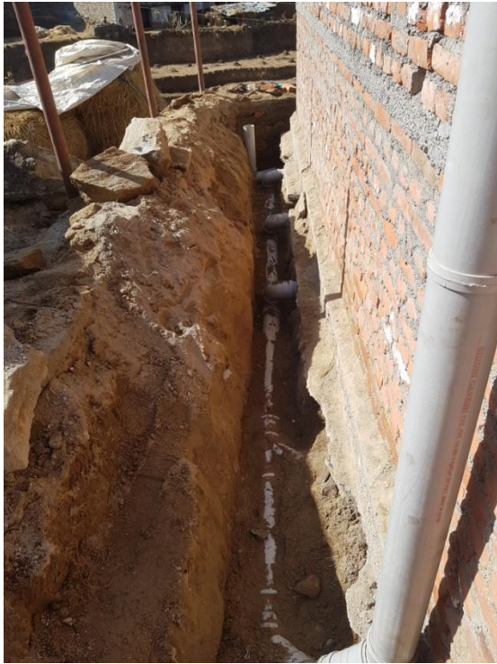
Vent pipe and drainage at upper toilet.
