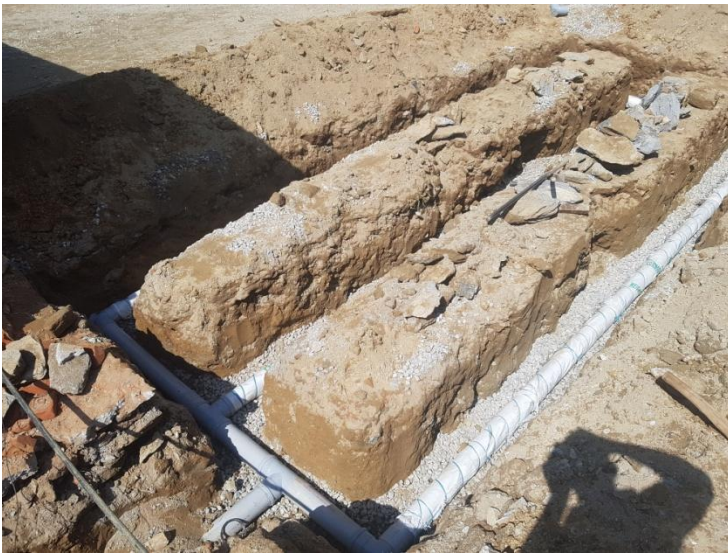
Laying of perforated & fabricated PVC pipes.
