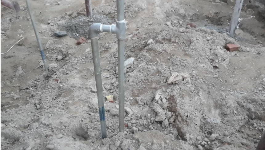
Water filler pipe line for both upper and lower tank.
