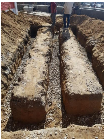
The soakage PVC pipes are covered and filled with gravel.
