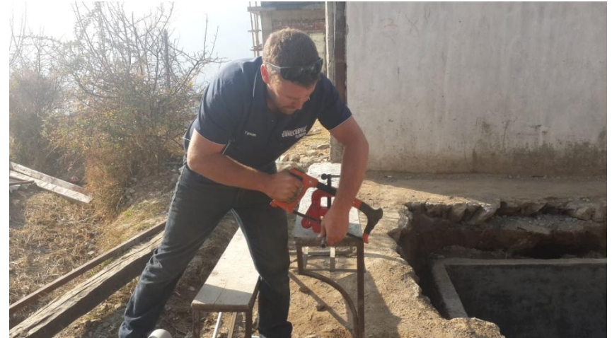
GI pipe works – for the tap connections.
