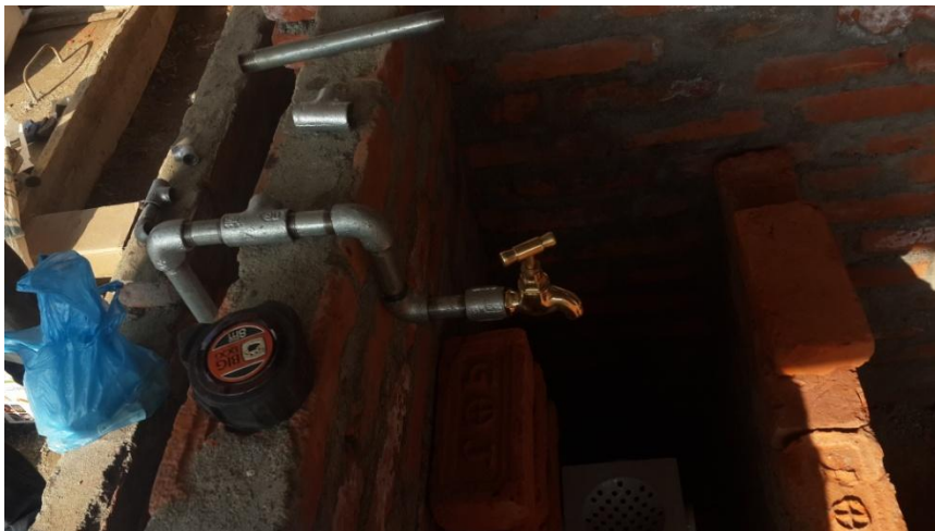
Hand washing and water drinking taps for lower toilet.
