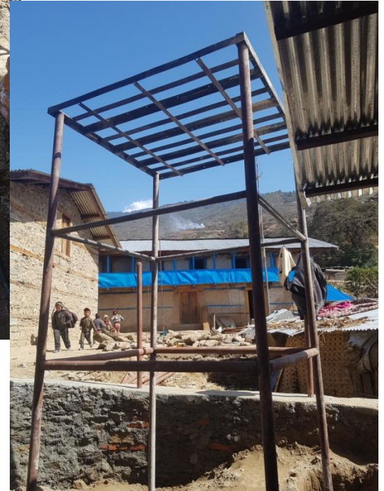
New water tank stand placed beside upper toilet
