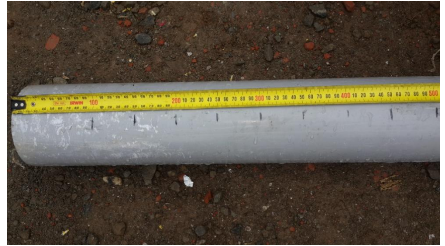
Marking at 2 inch distance to make a hole on 4 inch PVC pipe to be used for soaking trench.
