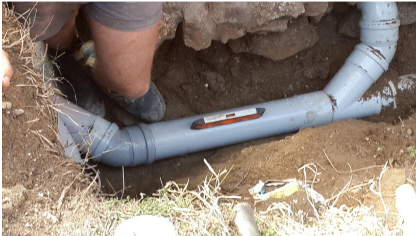
Drainage systems connected to septic tank of lower toilet.
