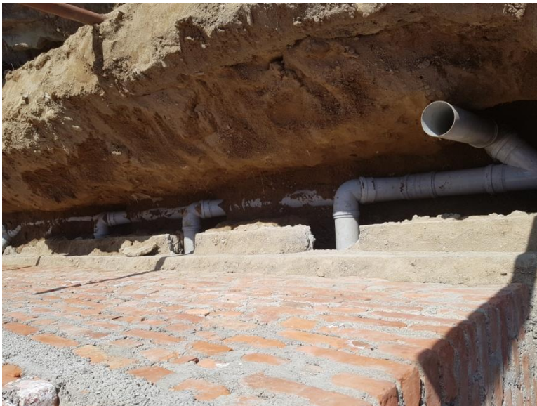
Toilet pan setting, drainage and vent pipe at upper toilet.
