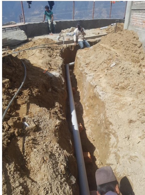
Drainage from septic to soakage trench – upper toilet
