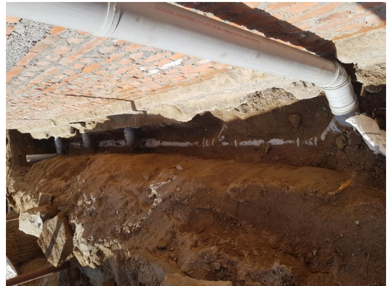
Toilet pan setting, drainage and vent pipe at upper toilet.
