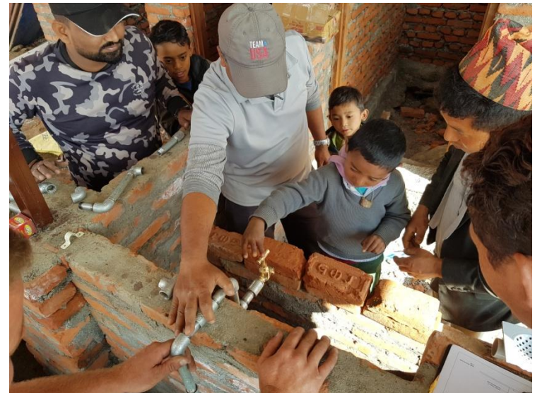
Checking the tap height by using lower class children – lower Toilet.
