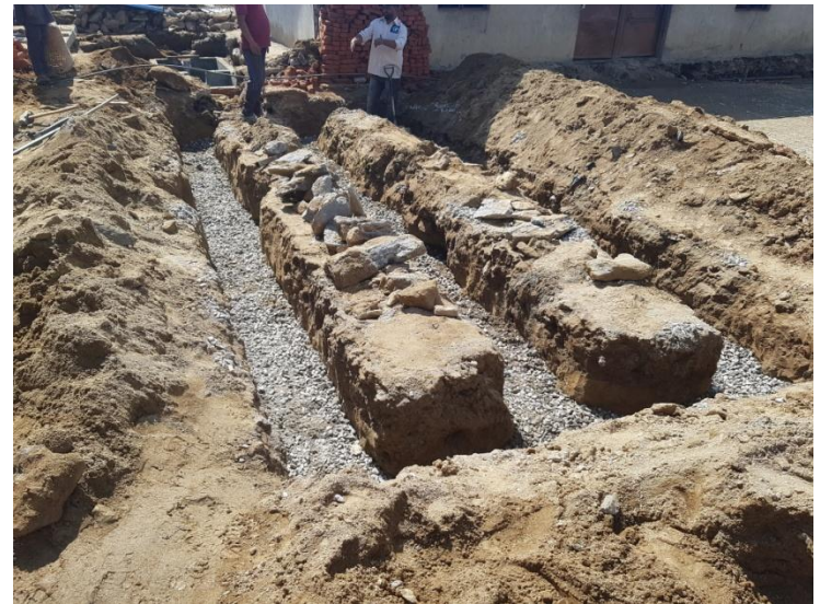
Covering of the Pipes by gravel up to 6 inches above from pipe and covered the trench by soil on top.
