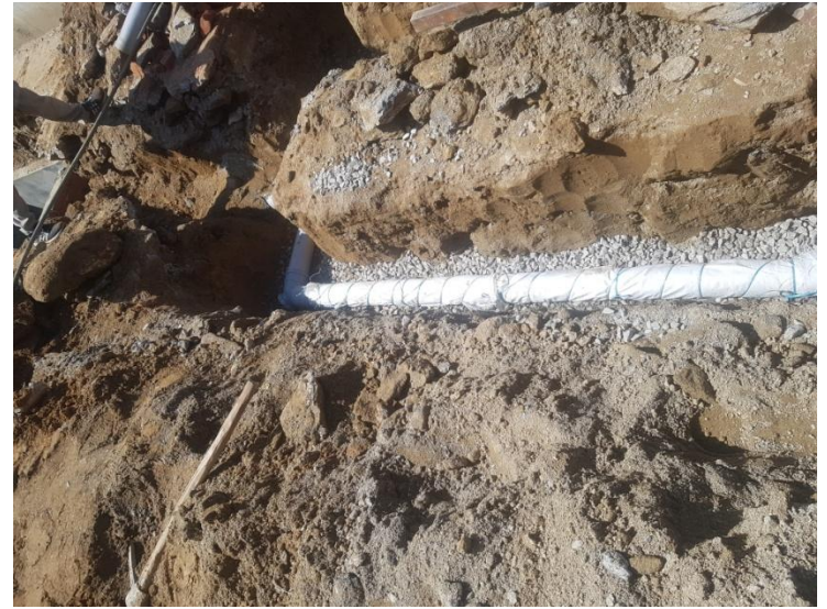
The trench is filled with gravel up 9 inch from bottom.
