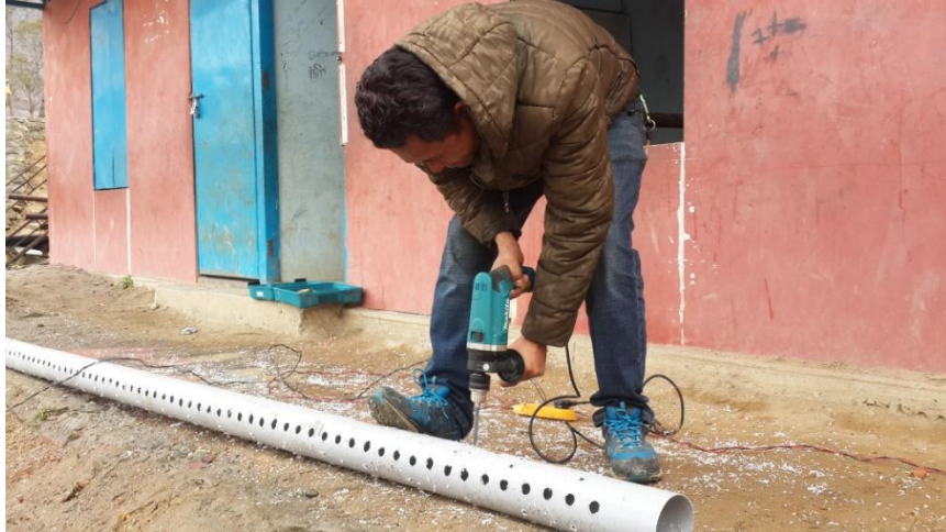
Making a hole on 4 inch PVC pipe.
