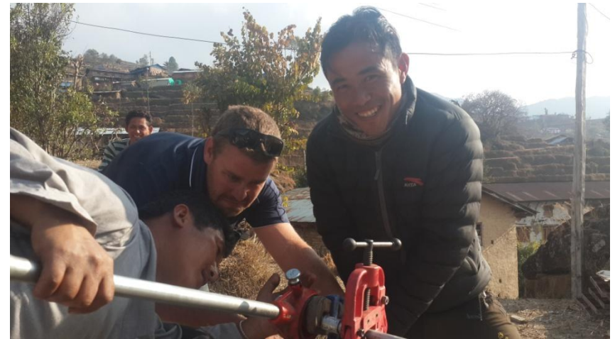
The SMC chairperson Suke Tamang enjoying by making thread on the GI pipe.
