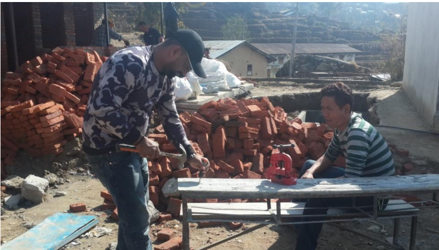
Fixing the GI threader
