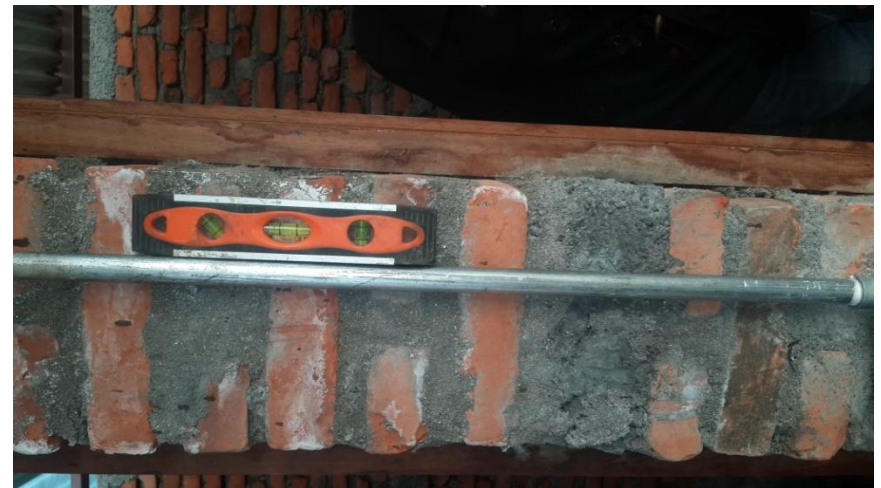
Pipe level checking
