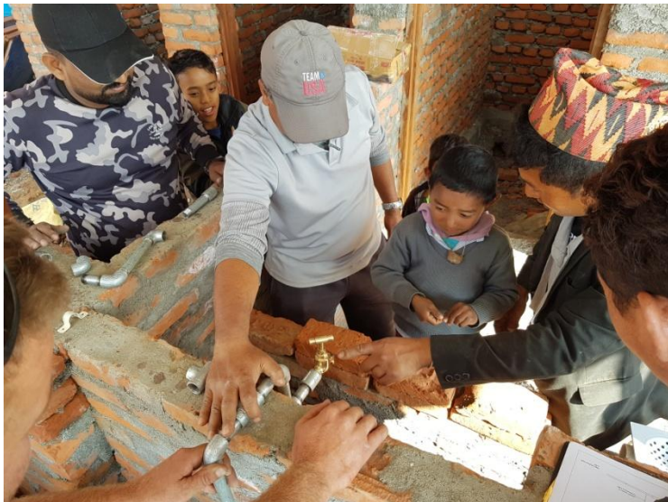
Checking the tap height by using lower class children – lower Toilet.
