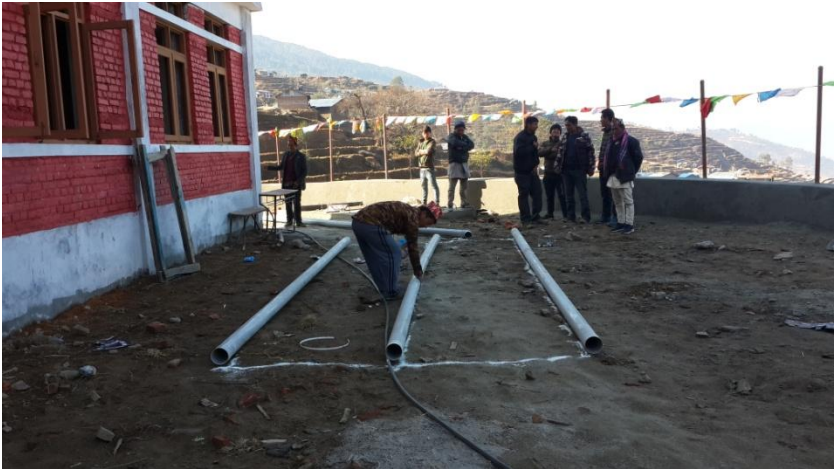
Soakage trench marking for upper toilet.
