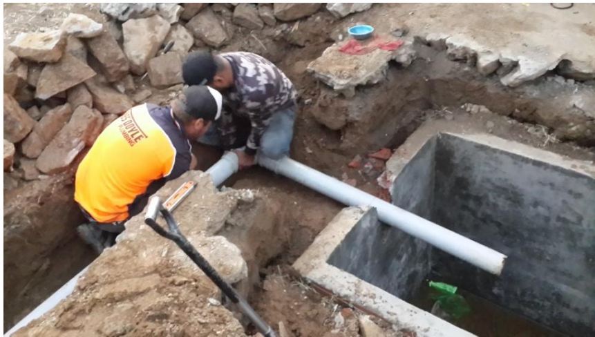
Drainage from the toilet, hand washing and drinking water taps to the septic tank at lower toilet.
