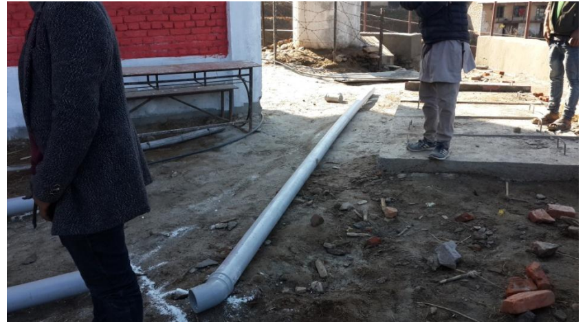
Soakage trench marking for upper toilet.
