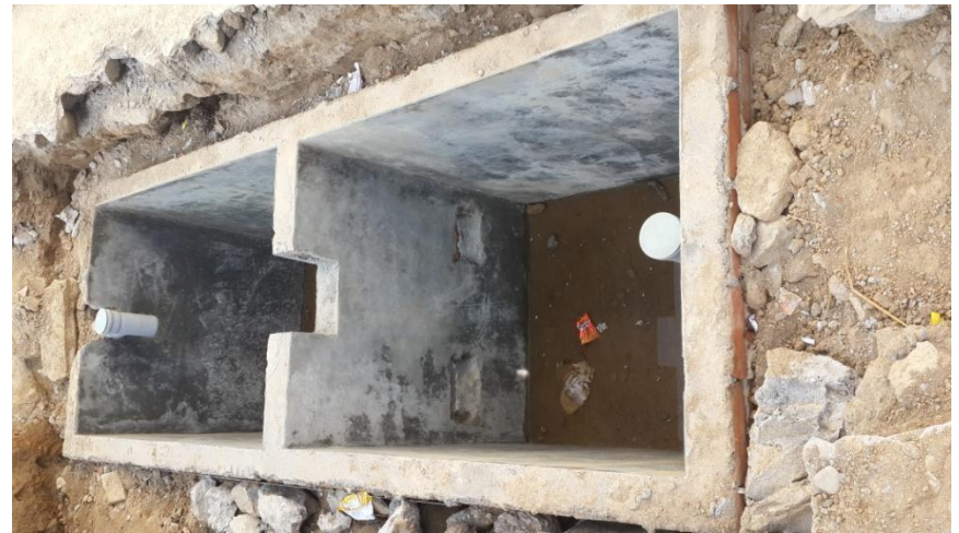
Drainage from the toilet, hand washing and drinking water taps to the septic tank at lower toilet.
