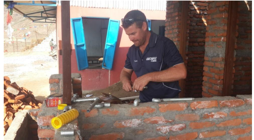
Tyson Knight – working on GI connectors.
