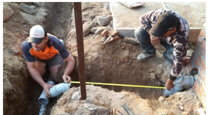
Drainage systems connected to septic tank of lower toilet.
