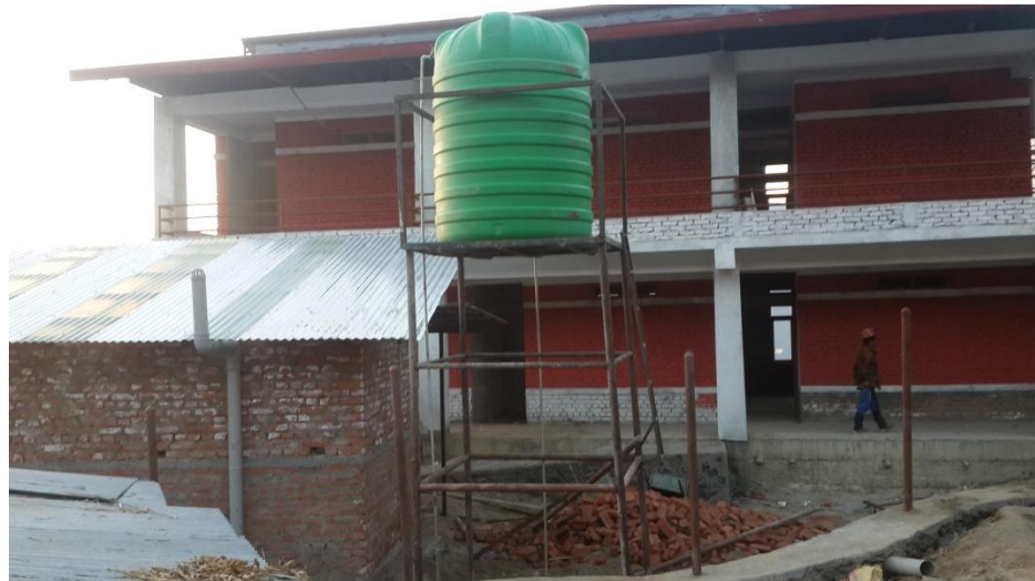
New water tank installation and the water line is connected to the upper toilet, hand washing and drinking taps as well as connected to the lower toilet.
