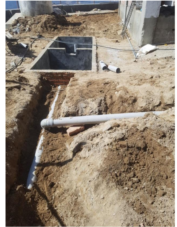
Drainage from toilet and hand basins to septic tank at upper toilet.
