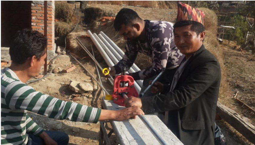
GI pipe works – for the tap connections.
