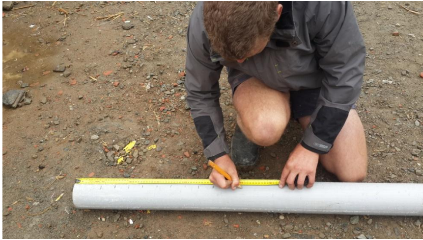
Marking at 2 inch distance to make a hole on 4 inch PVC pipe to be used for soaking trench.
