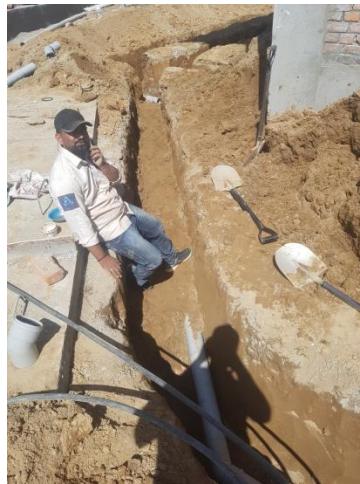
Drainage Pipe line to soakage trench.
