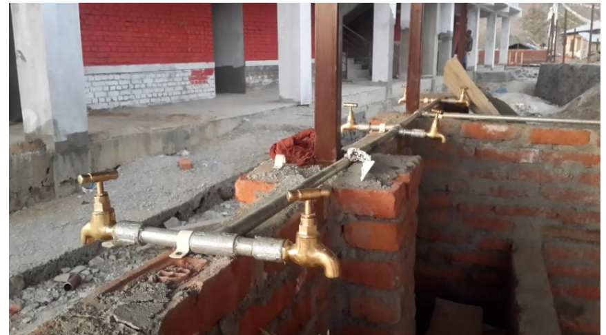
Inside & out side tap connections.
