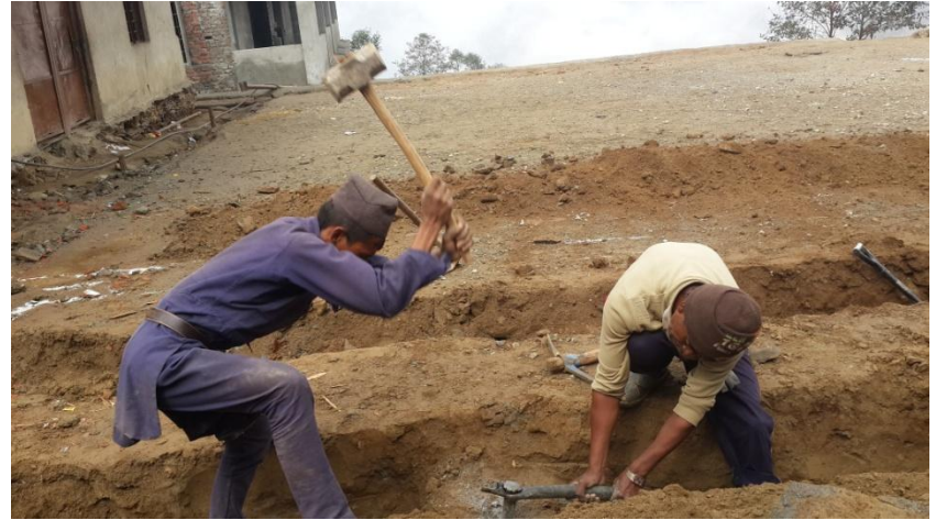
Marking and soil excavation work for SOAKAGE TRENCH – for Lower toilet.
