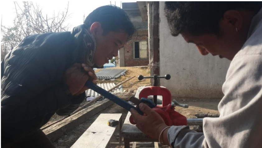
The SMC chairperson Suke Tamang enjoying by making thread on the GI pipe.
