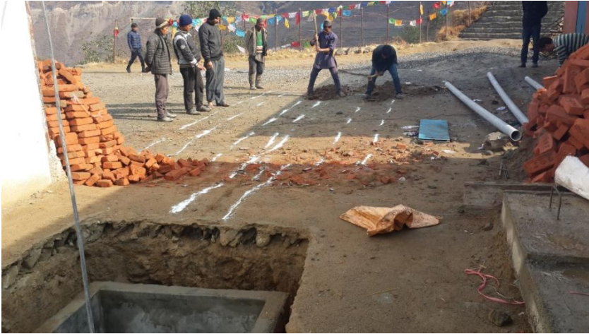
Marking and soil excavation work for SOAKAGE TRENCH – for Lower toilet.
