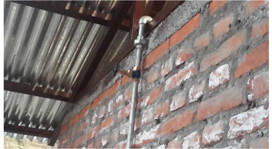
Pipe line and gate valve to toilet block – upper toilet.
