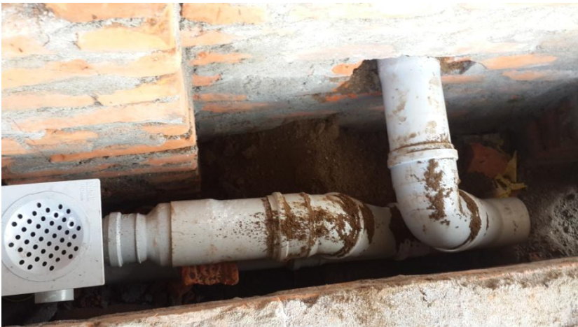
Drainage work for hand washing and water drinking taps.
