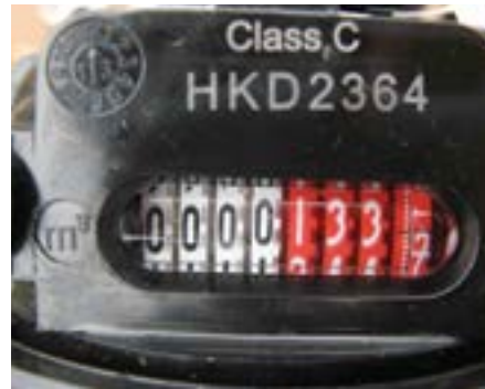
FIGURES 23: Water metres were installed (which required new galvanised pipes due to deterioration) and systems for regular readings were established.
