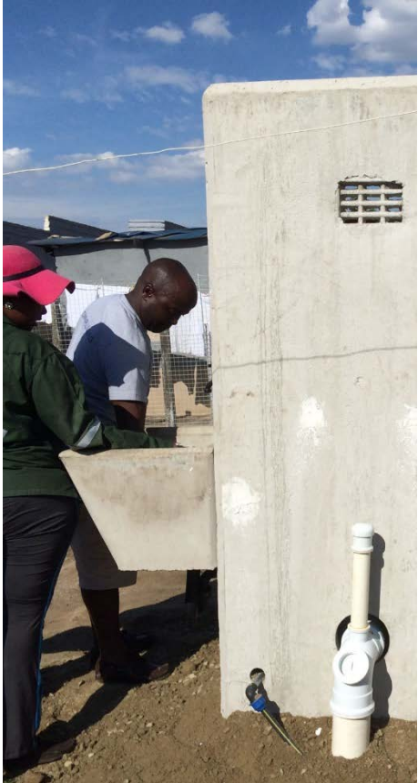
The completed toilets are connected, and tested for leaks
