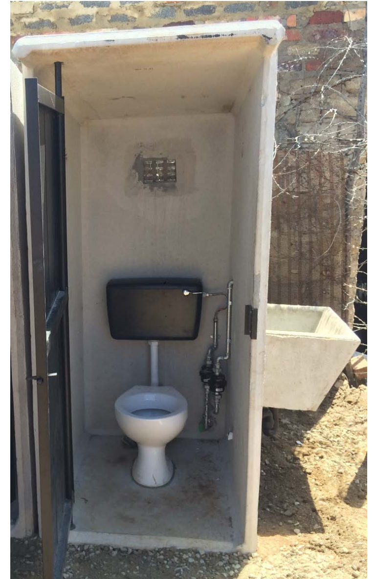
On completion gravel is compacted around the edges of the toilets to improve access, and ensure storm water flows away from the toilets
