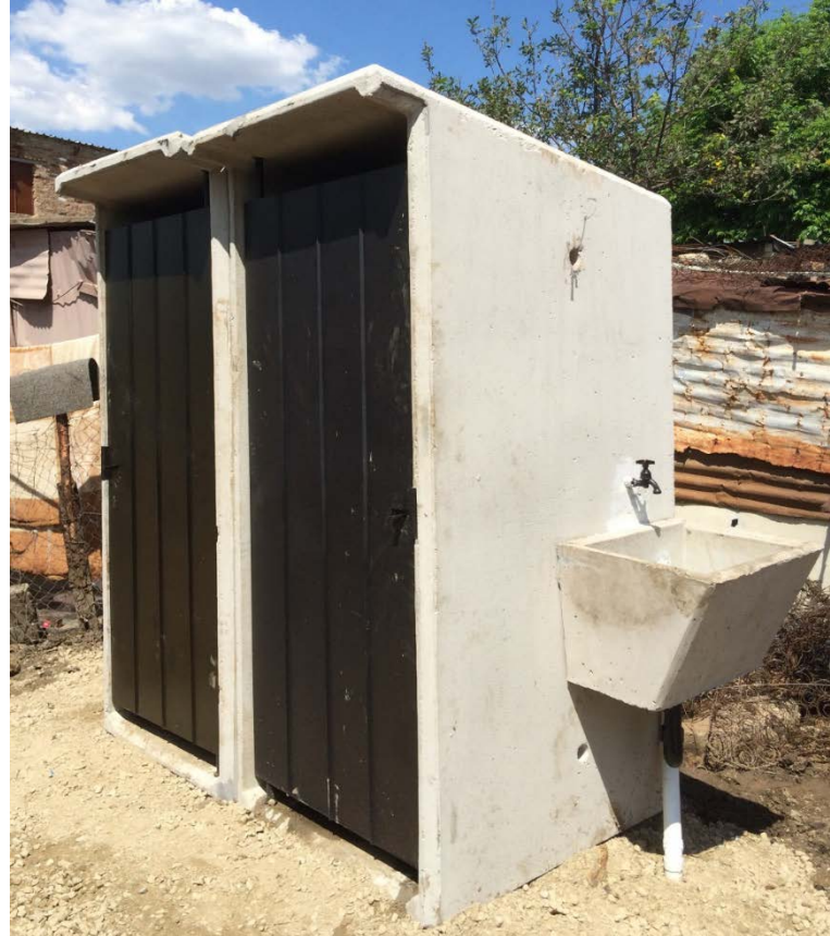
On completion gravel is compacted around the edges of the toilets to improve access, and ensure storm water flows away from the toilets
