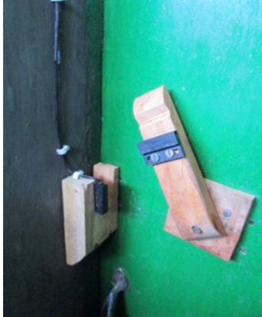
The inside lock in the open position but the door is secured externally to prevent access by young children and animals
