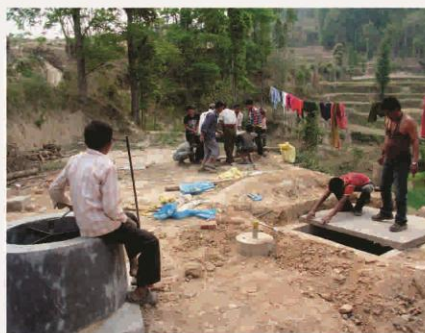
21. Closing of septic tank and bio gas outlet.
