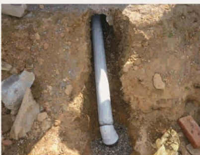
16. Biogas plumbing and toilet pan insertion work.
