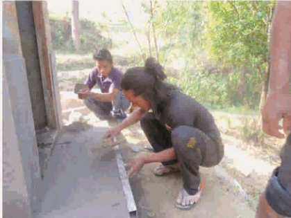
17. Plaster and toilet step slab preparation work..
