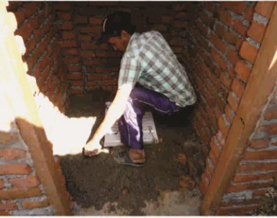
15. Septic water treatment system and toilet pan insertion work.
