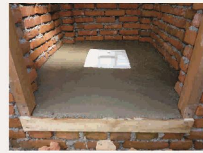
15. Septic water treatment system and toilet pan insertion work.
