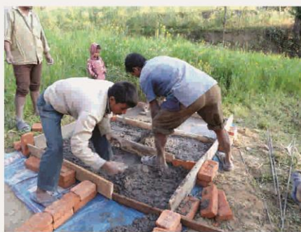
7. Bio gas DOM & SLAB preparation.
