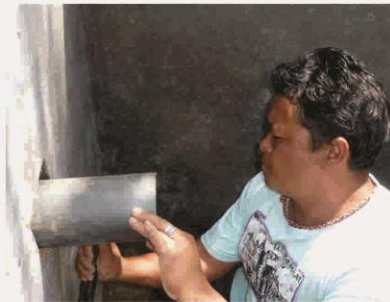
14. Plumbing works and toilet pan insertion.
