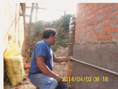
18.GI Tap pipe work- for inside and out side tap .
