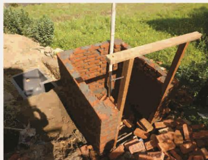
9. Door frame placement and wall work.
