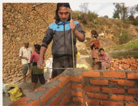
10. Roof hooking rod insertion and toilet wall work.
