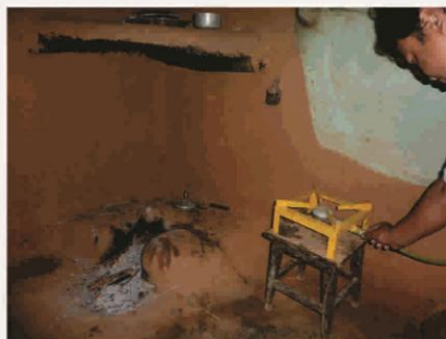
19. Biogas mixture, pipe line fitting and stove fitting. .
